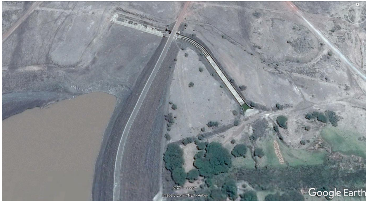
Figure 3.21: Melka Wakena dam and Spillway
