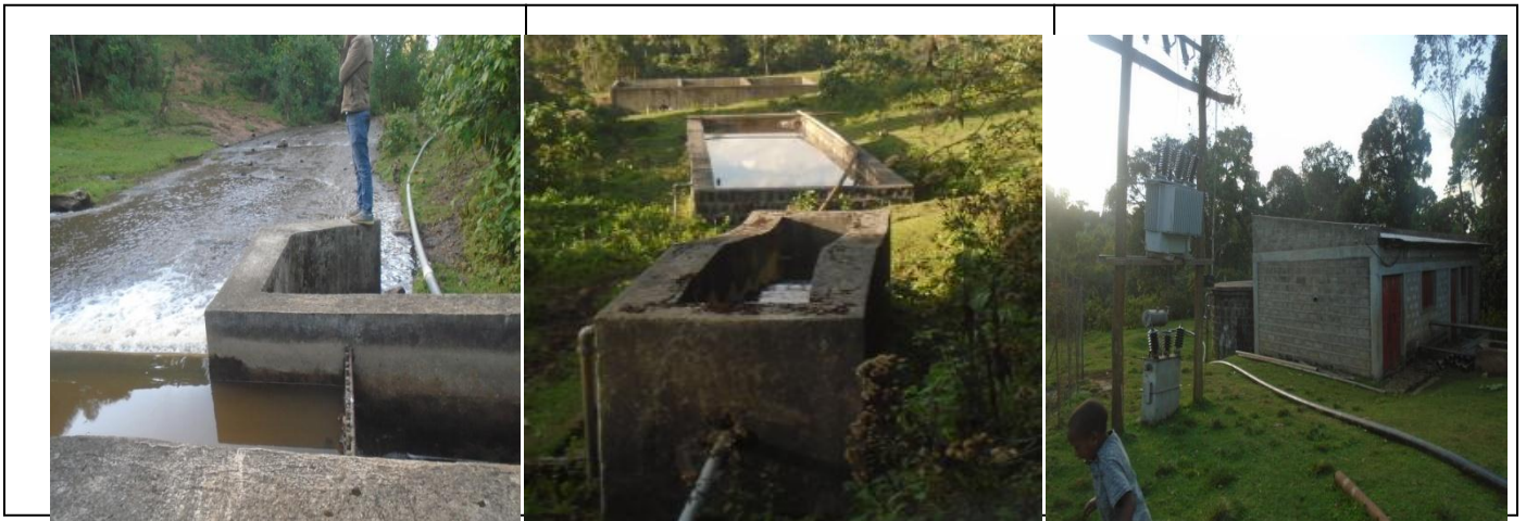
Figure 3-2: Image of existing Masha town water treatment plant, intake and wet well
