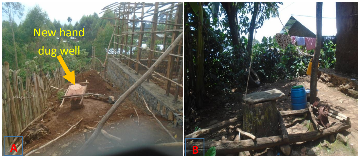
Figure 4-5: Image showing appearance of hand dug newly constructed (A) older wells (B)
