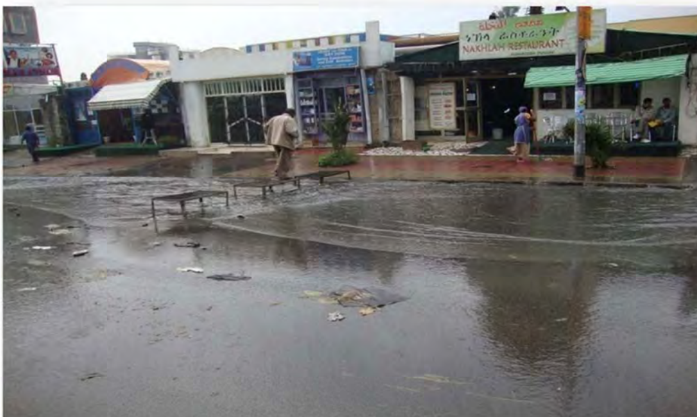
Fig 1.4) Drainage problem at Ring road
