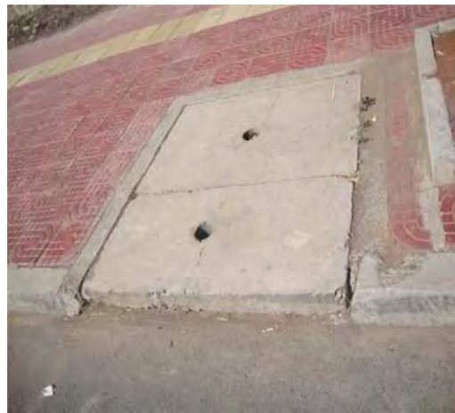
Fig 3.5 b) Inlet cover overlapped with the Pavement (no opening at all)
