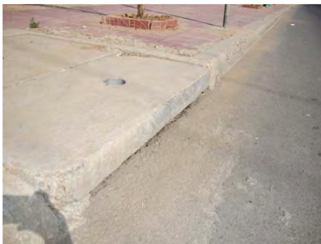
Fig 3.5 c) under designed curb height (12 cm) and small inlet opening
