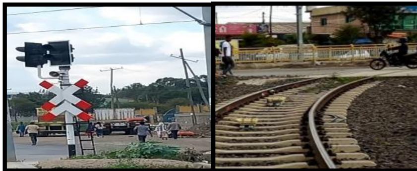
Figure 4.13: Level crossing at AALRT Kality
