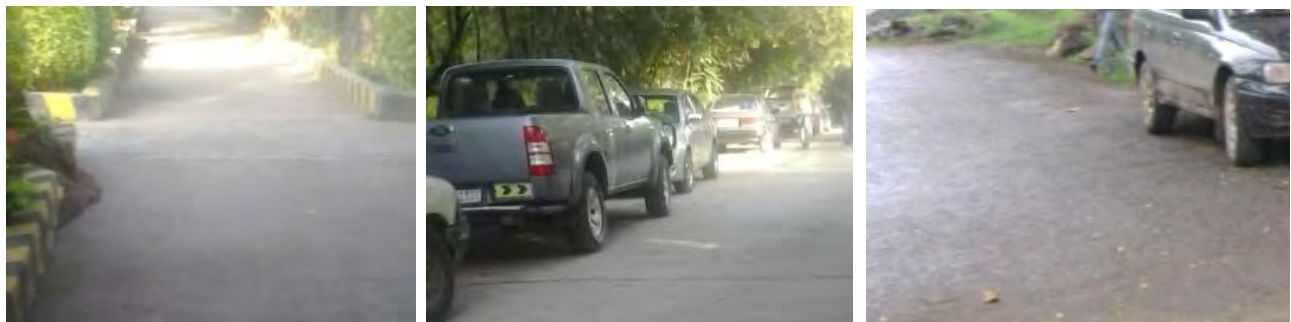
Figure 37. Existing Asphalt and concrete paved street surfaces (Photos by author)
