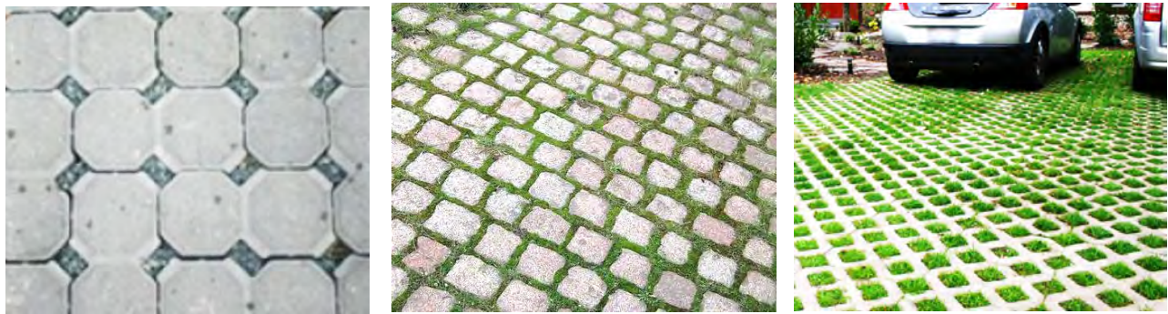
Figure 38. Permeable pavement patterns (source; Pinterest images)
