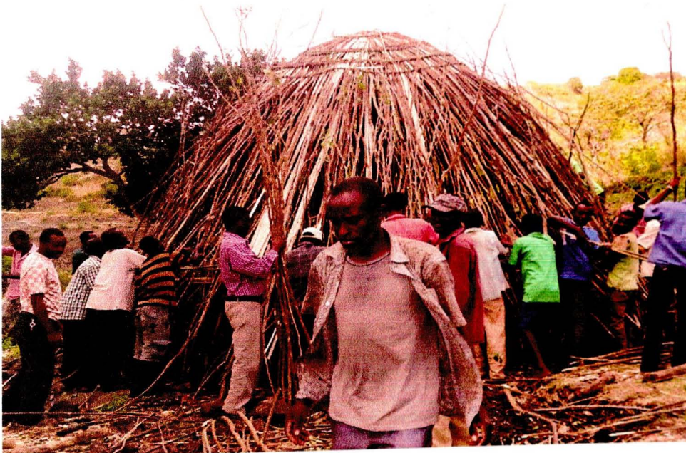
Dhele Idir association including: mala , lathi and ayle , constructing a house for mala widow in April 2013
