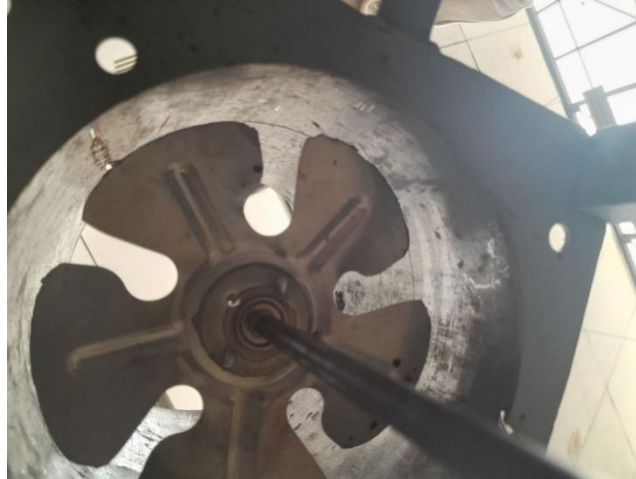
Figure 3.3.4 Turbine installation at the bottom of chimney
