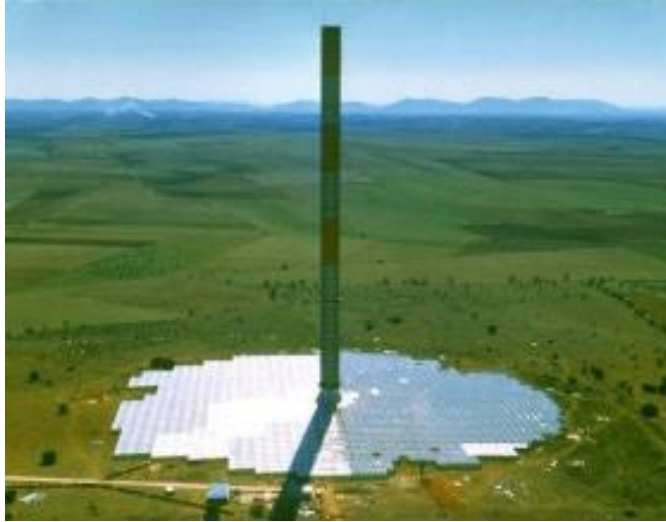
Figure 1.1 First solar chimney power plant prototype in Manzanres [3]
