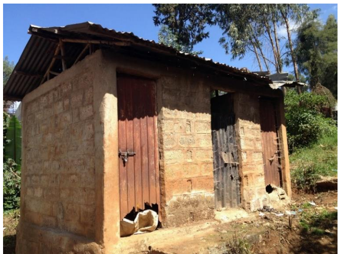
Pic 4. Public Toilet Woreda 5
