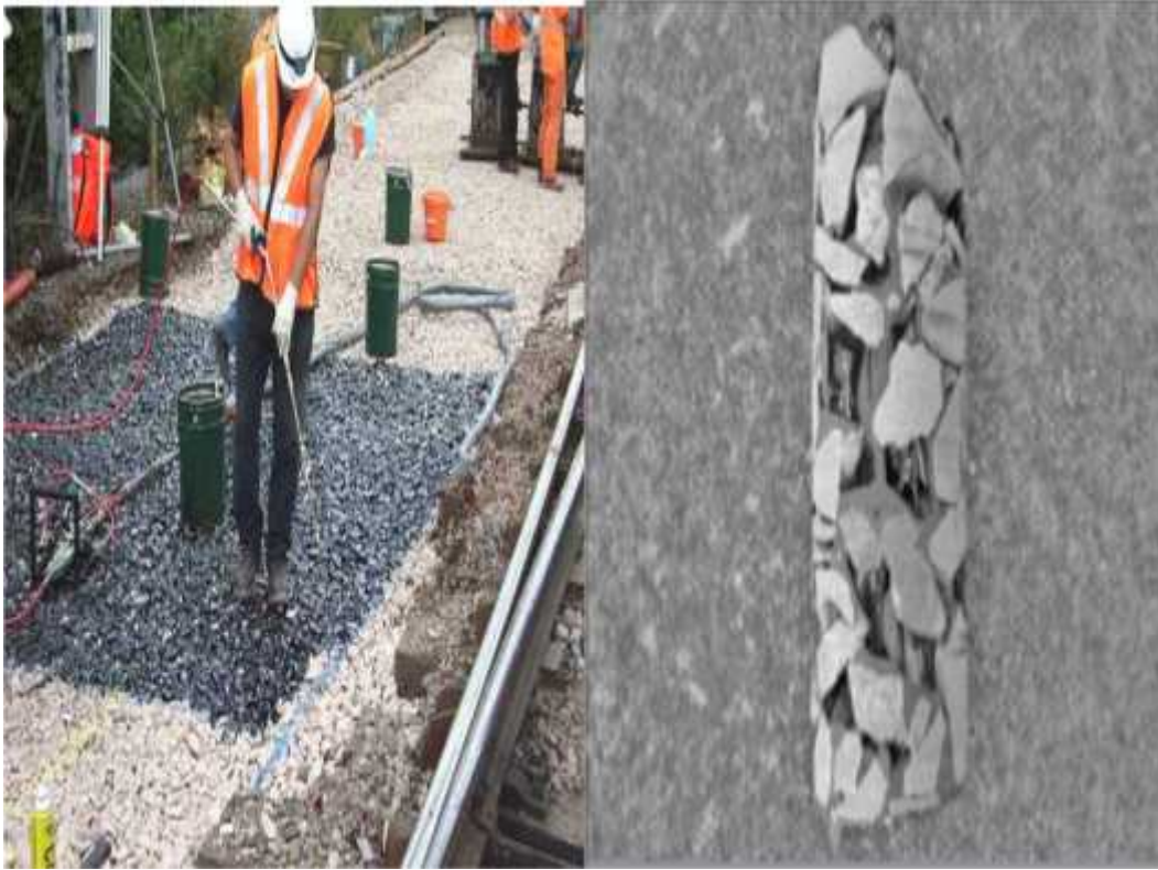
Figure 9: Close view of XiTrack Stabilized railroad ballast (woodward et al, 2007)
