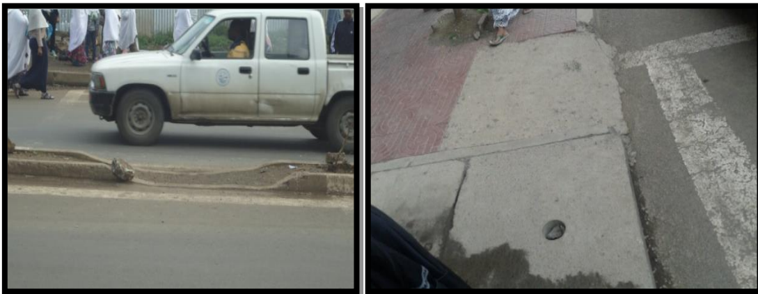
Figure 4-5: Comfortable crossing at median for wheelchair users as well as other physically disable
