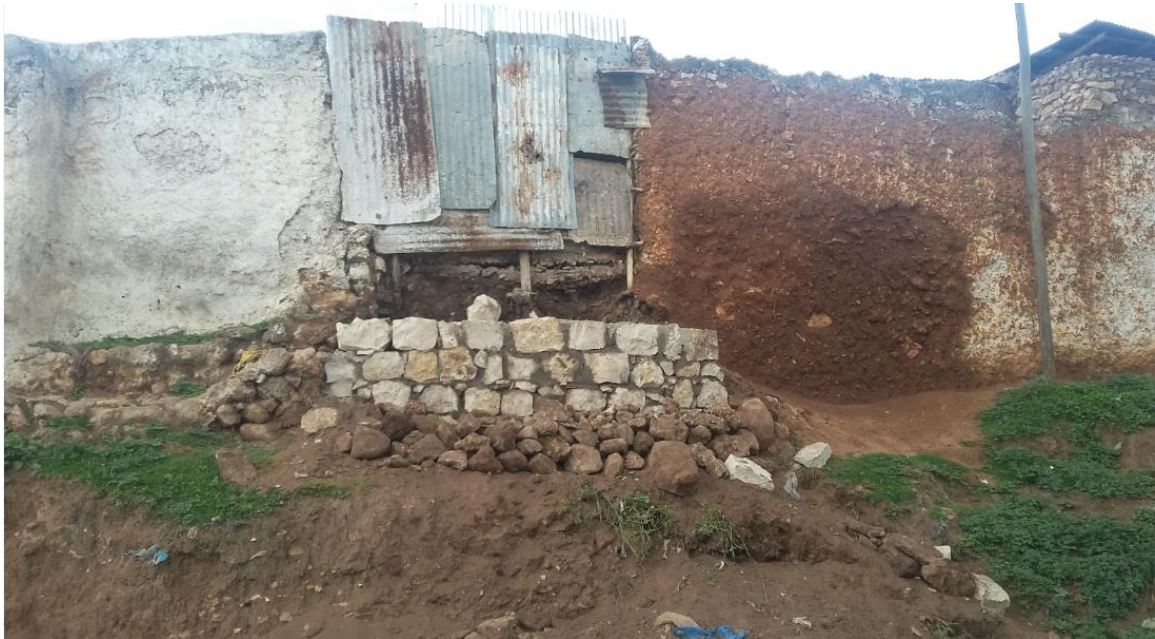
Figure 36. Rebuilding the demolished part of Jugol wall (Sources: The Researcher, 2018)
