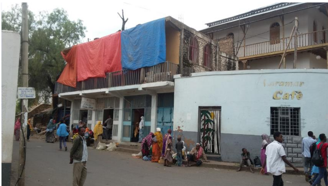
Figure 27. Illegal construction in the compound of Etege Menen (Sources: The Researcher, 2018)
