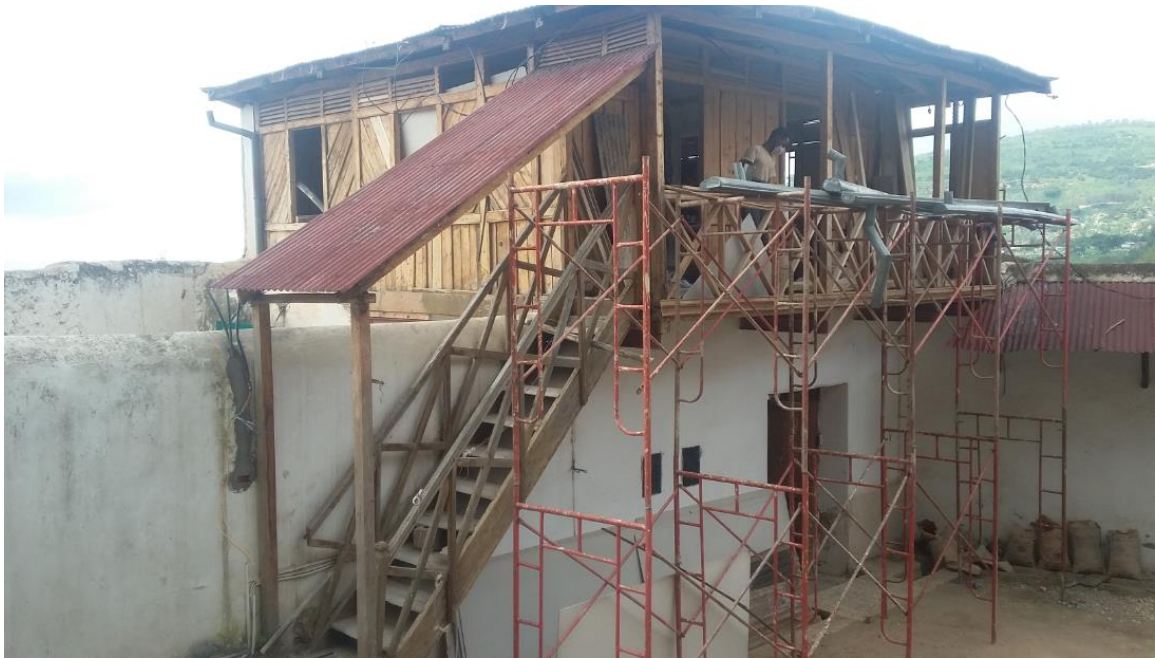
Figure 14. The Bridge house (Sources: The Researcher, 2018)
