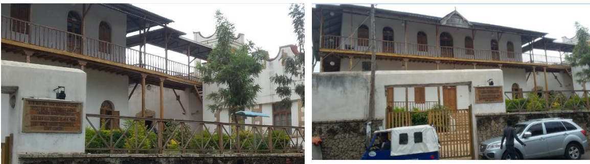
Figure 21. Post restoration of Etege Menen house (Sources: The Researcher, 2018)
