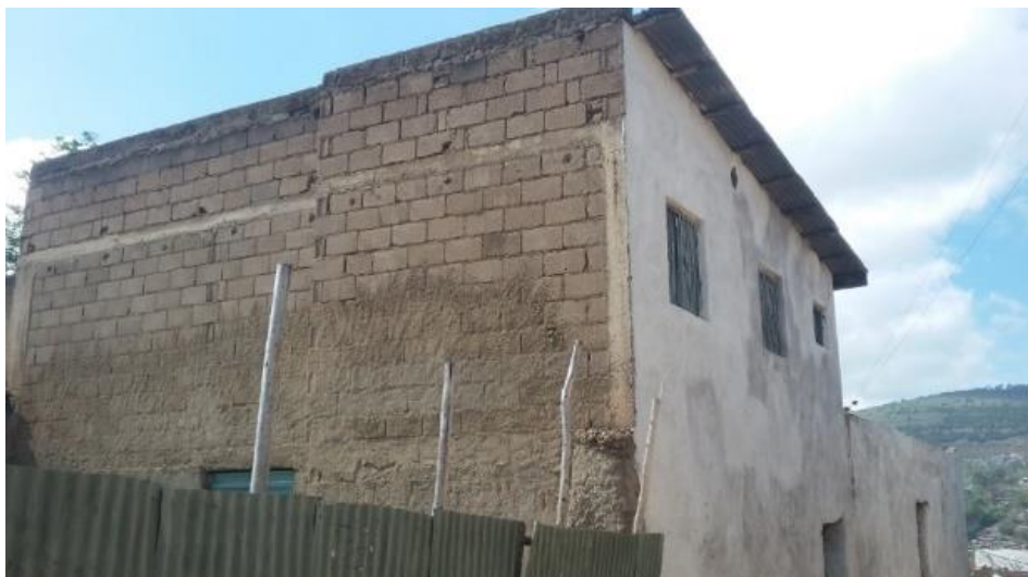
Figure 28. Building constructed using HCB and cement plaster (Sources: The Researcher, 2018)
