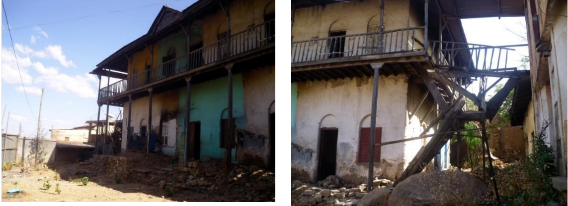
Figure 20. Condition of the building prior to restoration (Source: JHCO,2018)
