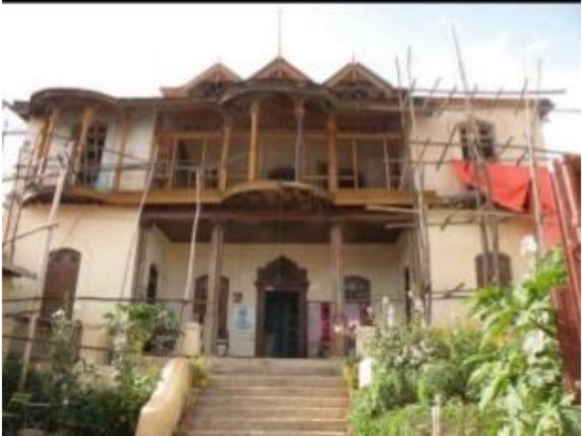
Figure 16: Ras Teferi house during restoration (Source: Hisham M, 2010)
