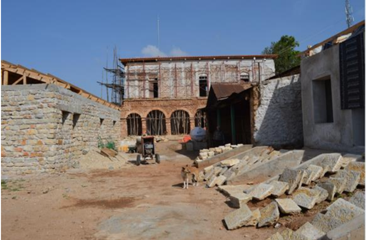
Figure 24. During restoration work (Source: JHCO, 2018)
