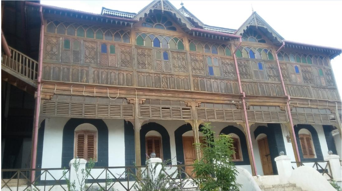
Figure 13. Rimbaud house after restoration (Sources: The Researcher, 2018)
