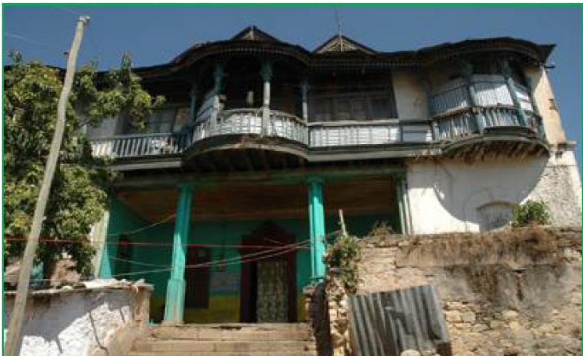
Figure 15. Prior restoration Tefari house (Source: Imran A., 2009)
