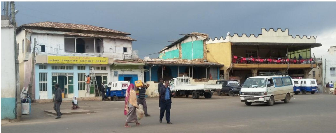
Figure 32. Partially demolished historic building. (Sources: The Researcher, 2018)
