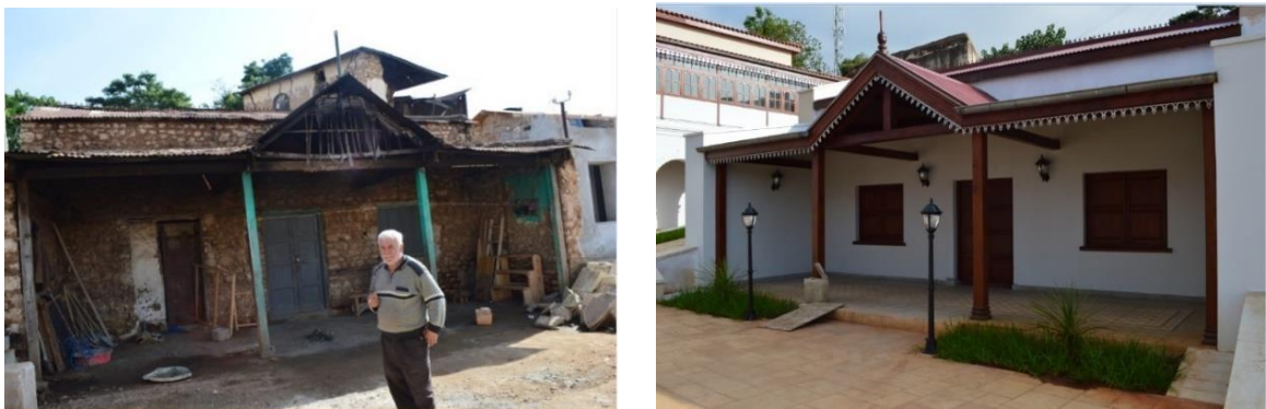
Figure 23. Prior & post restoration work
