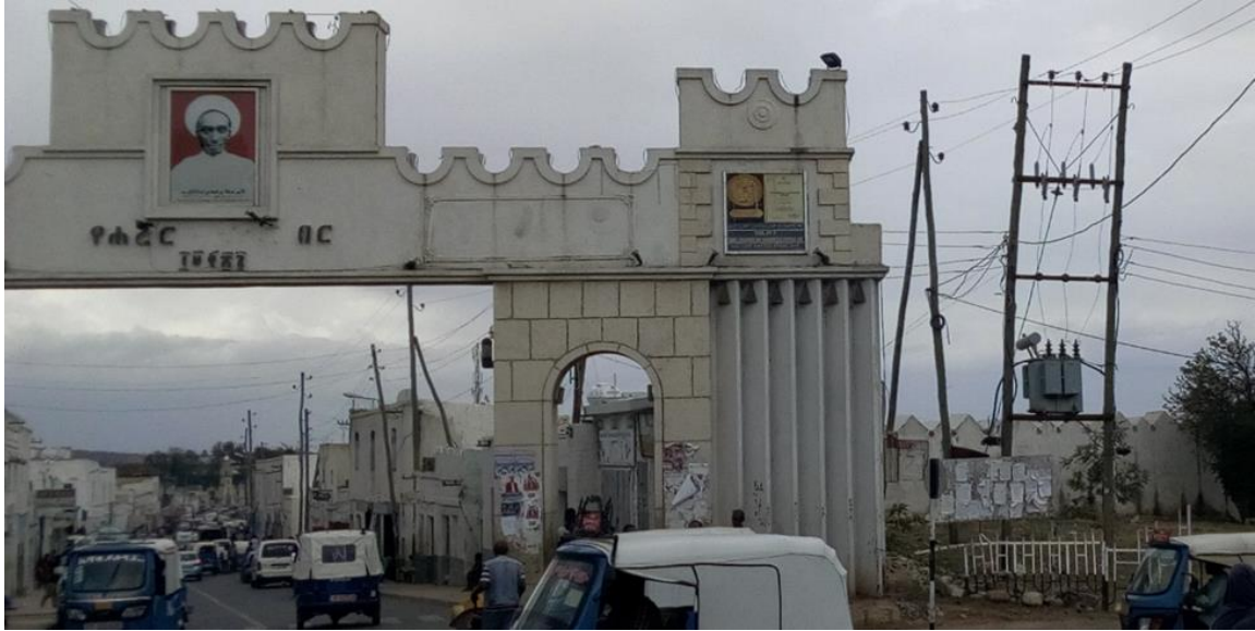
Figure 34. Distorted poles and cables of electrical installation
