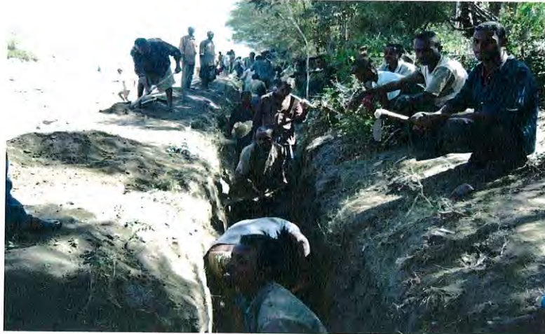
Figure 6 Community members participating in canal cleaning
