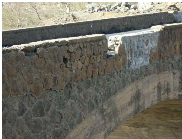
Figure 3-3 Reconstruction of the part of the parapet wall
