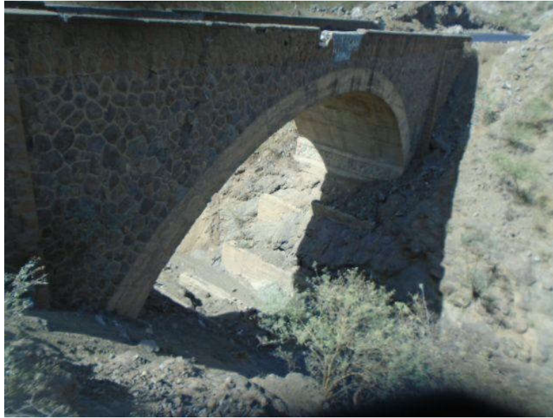
Figure 3-2 The Odie Bridge
