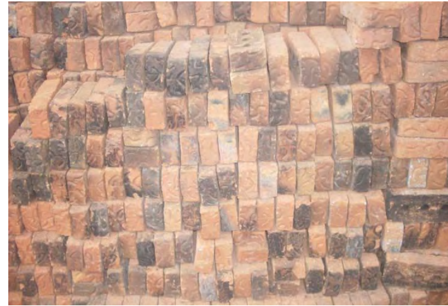
Photo-13 Over burnt clay bricks in Ethio brick factory.
