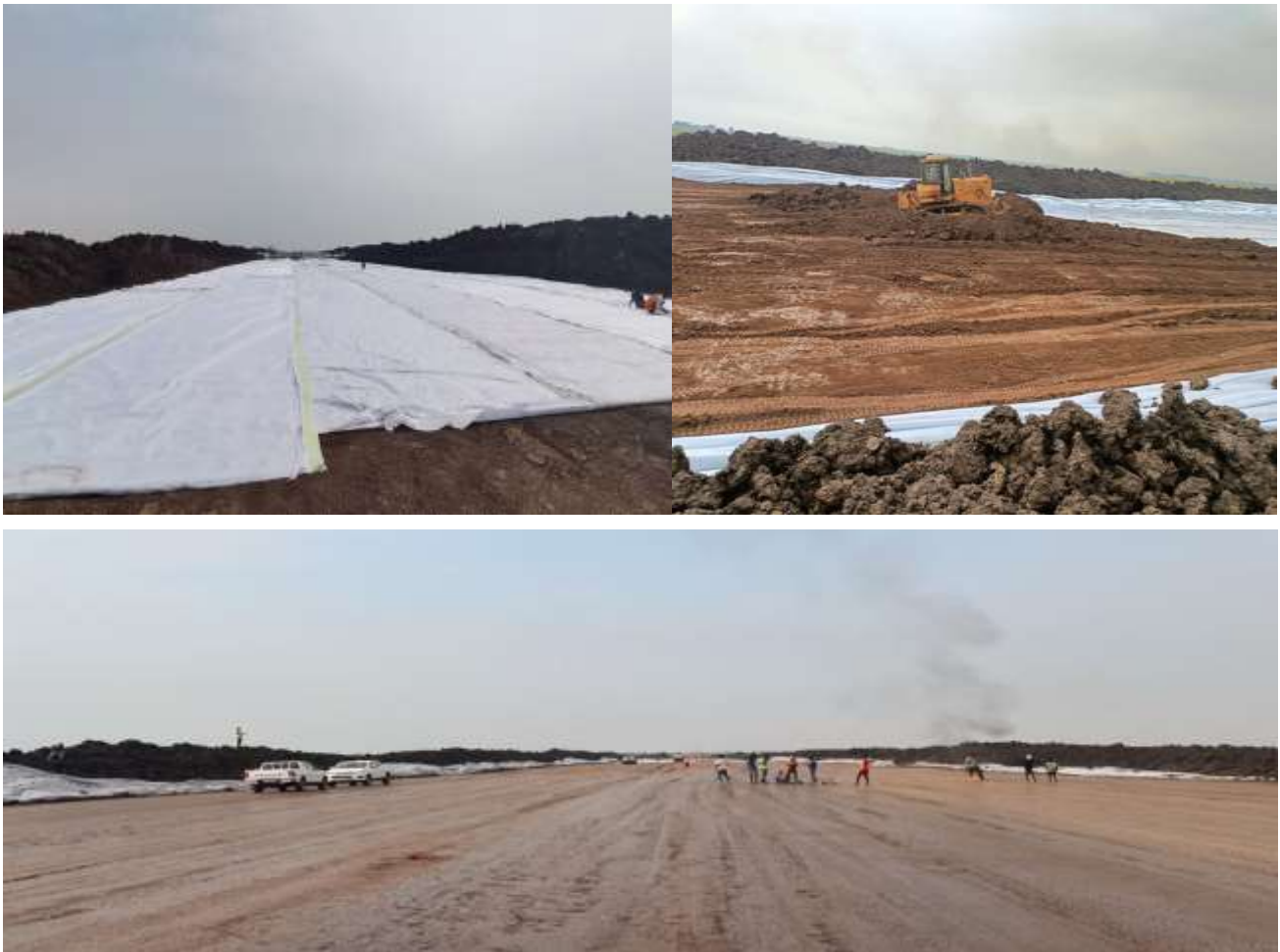
Figure 4-5: Embankment Construction using Geo-membrane in Project 2
