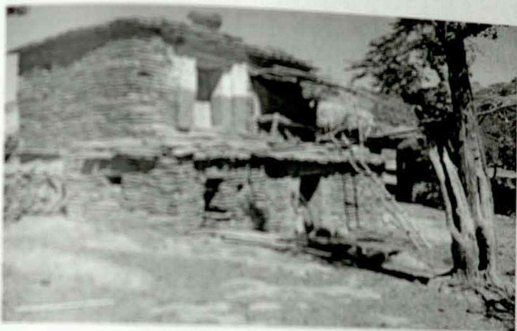
Plate VII: An Adirvashk with Stum and Soil Roof and a Gabek in the front underground
