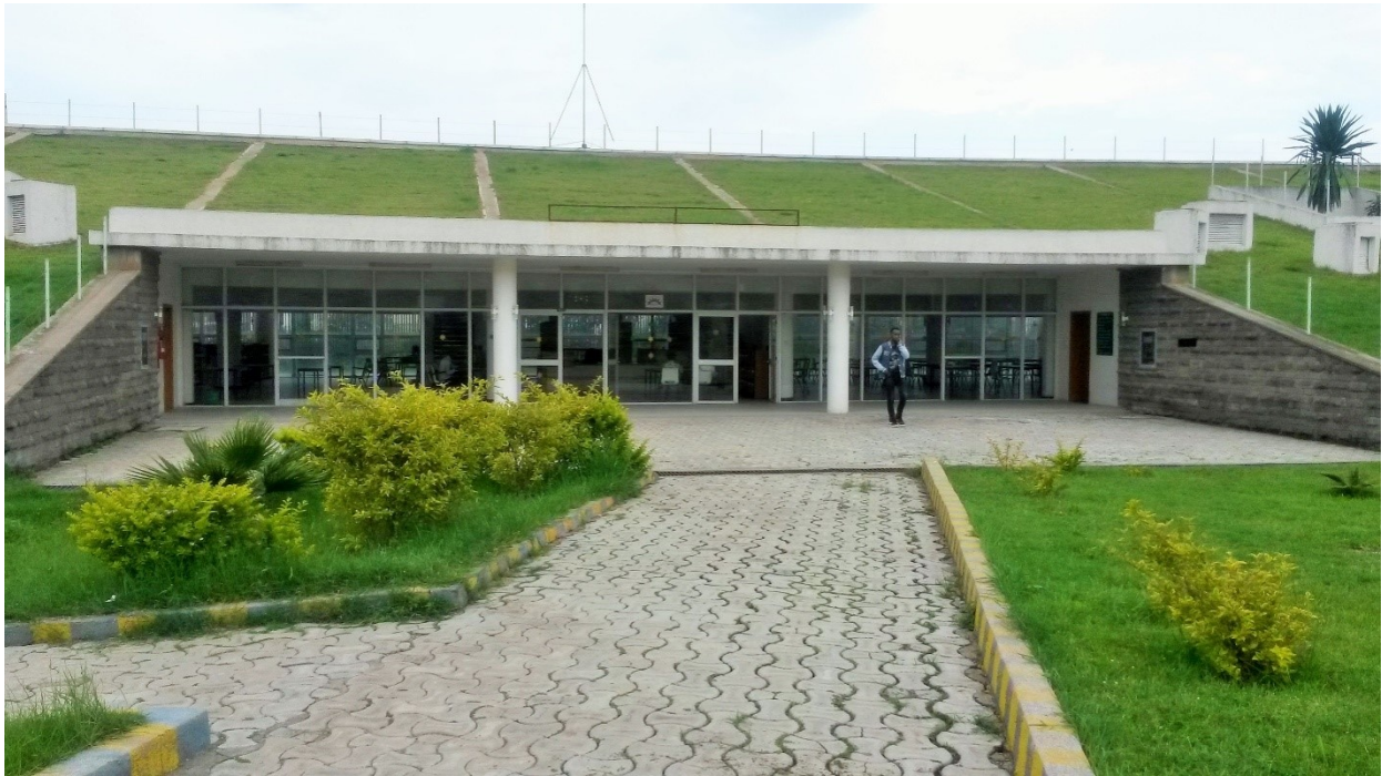
Figure 35 Front entrance to the library (in exceptionally good condition). Observe the sloping connections. Image source: site visit
