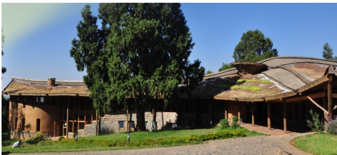
Figure 54 Exterior photo of Gulele Botanic Garden Center Extensive green roof after construction.
