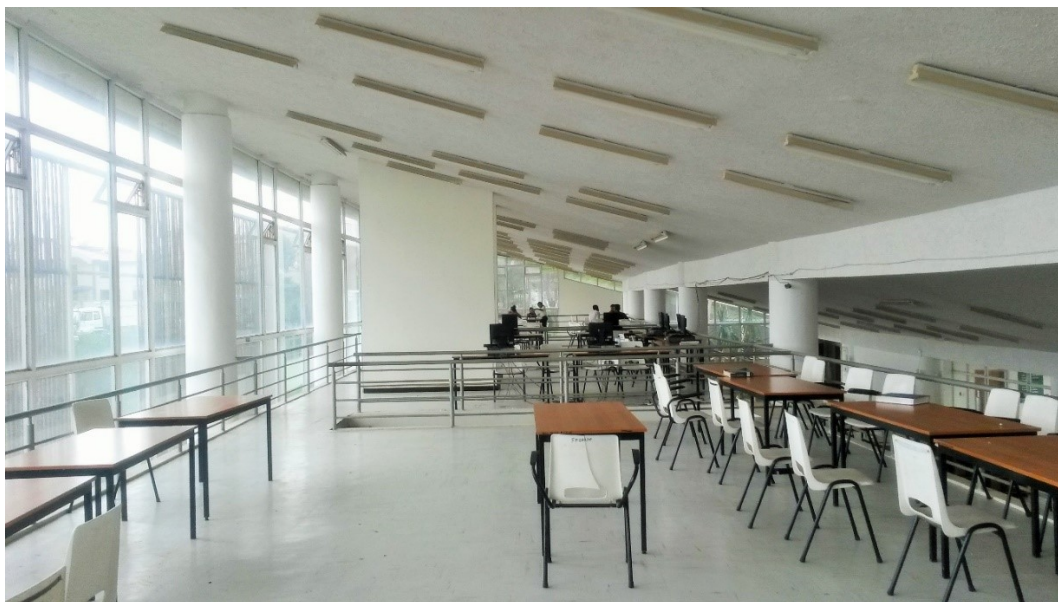
Figure 29 as we can see from these image, the reconstructed interior of the library has no leakage issues and being in very good and exceptional condition up to now. (Reading space). Image source: site visit
