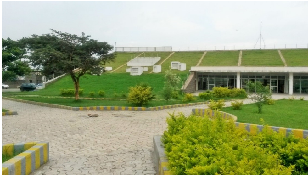
Figure 21 Current status of the green roof (right side, the reconstructed one, image source site visit
