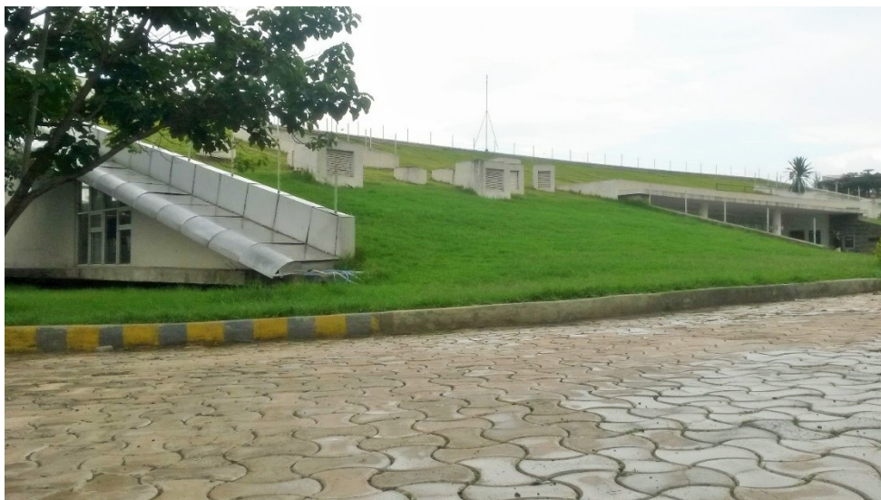
Figure 26 The Library seen from ant's eye view, connections and joints that need a specific design detail. Image source: site visit
