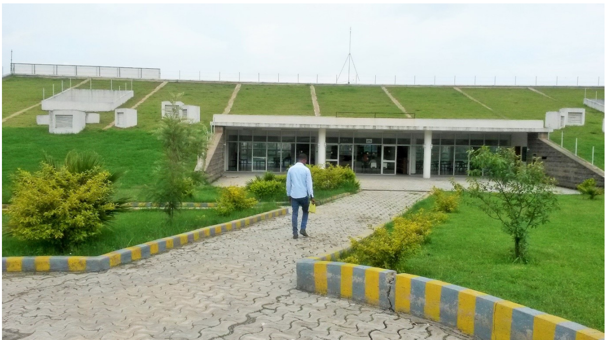
Figure 36 (View from the roundabout) Front entrance to the library (on exceptionally good condition) observe the sloping connections image source: site visit
