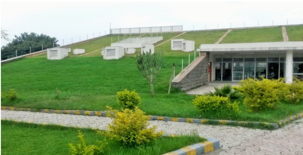
Figure 47 Hope university college library building green roof exterior view. Image source: site visit
