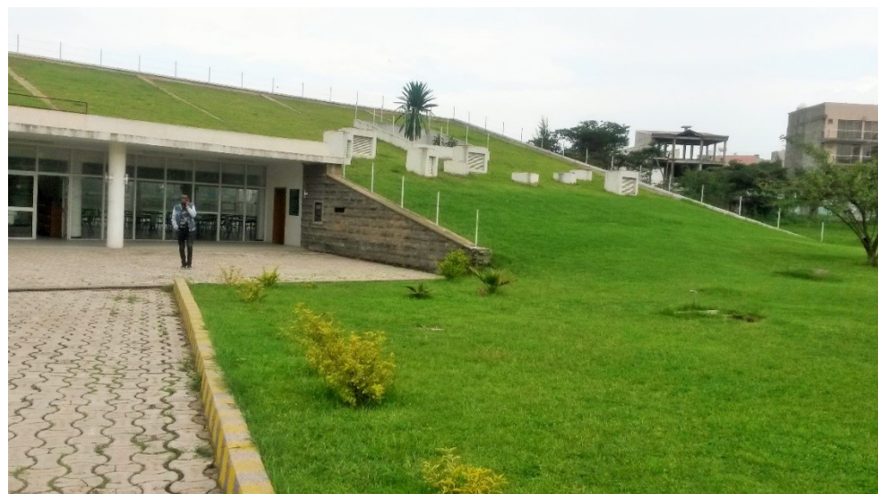
Figure 22the merging landscape with the surrounding Current status of the green roof (right side, the reconstructed one, image source: site visit
