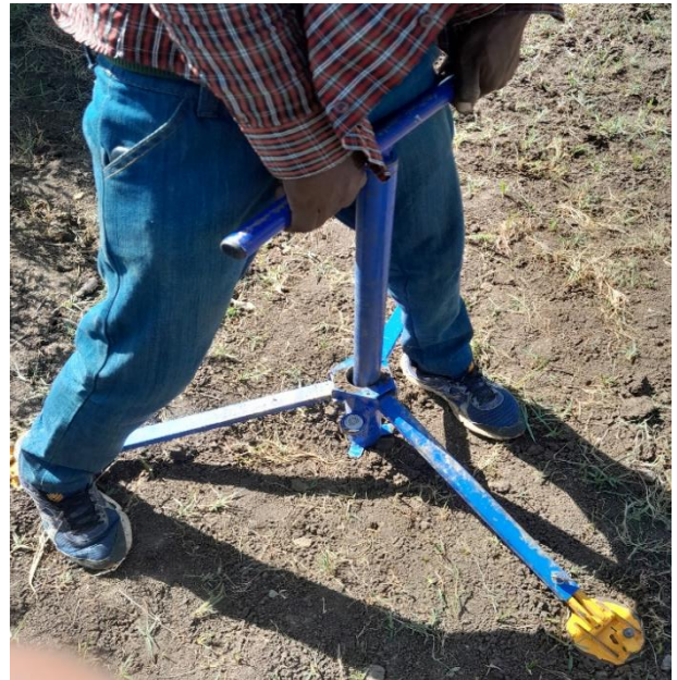
Figure 3-6 Installation of Access tubes
