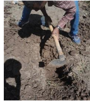
Figure 3-7 Digging Trench
