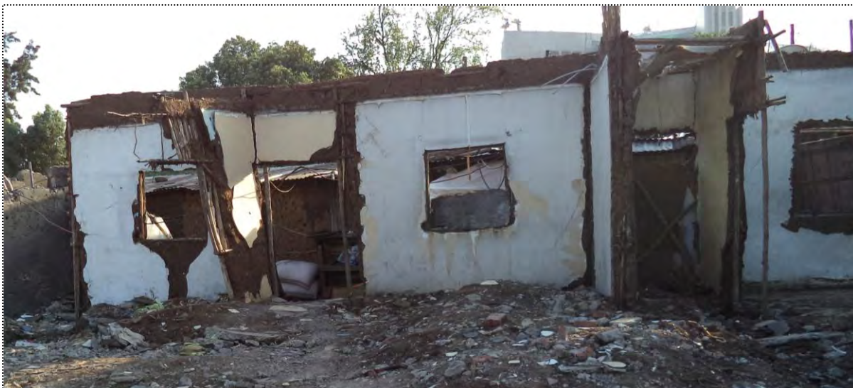
Figure 5.10: Demolition of non-structural buildings near to AU
