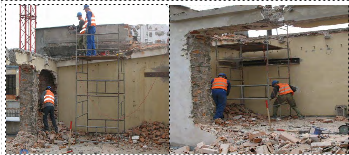
Figure 2.3: Manual demolition ( www.demolitionsquad.co.uk )
