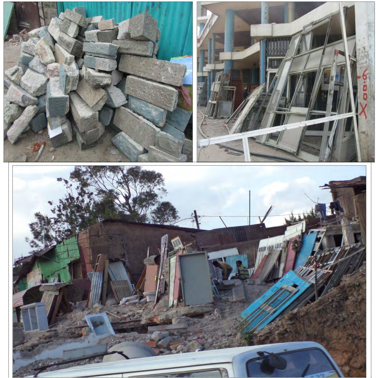
Figure 5.19: Dressed stone, windows and doors dismantled around legare and 22
