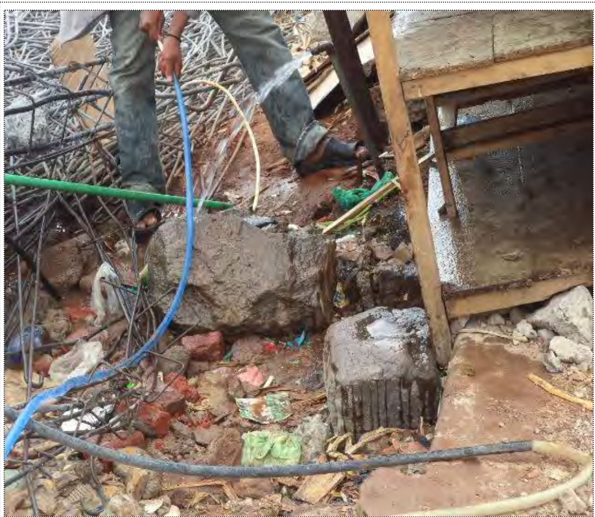
Figure 5.8: Demolition before water line service disconnected off ( American Gibi )
