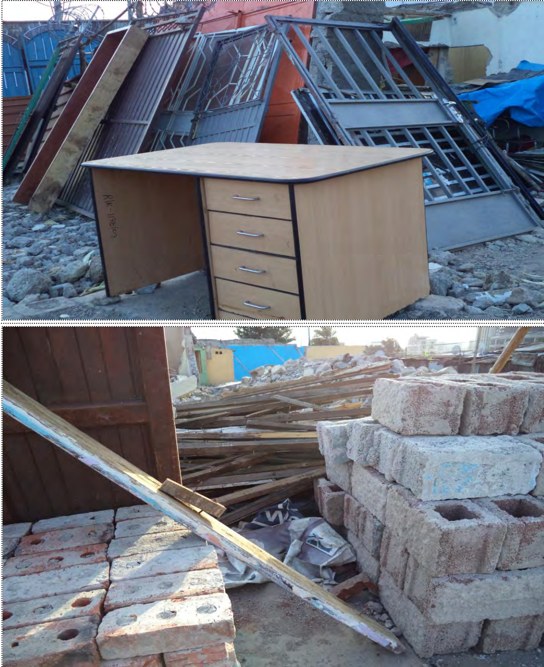
Figure 5.13: Dismantled doors, windows, bricks, HCB'S, and woods on site
