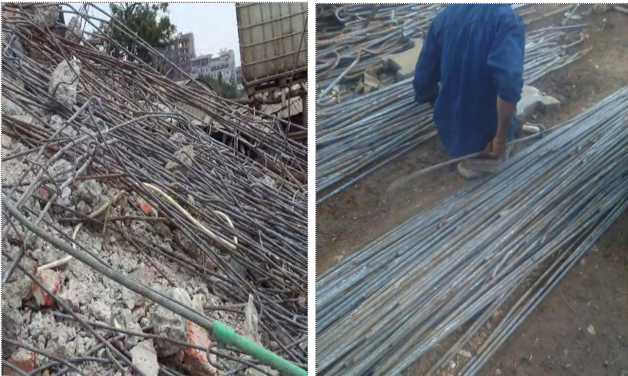
Figure 5.7: Steel bars after demolition of building components ( American Gibi )
