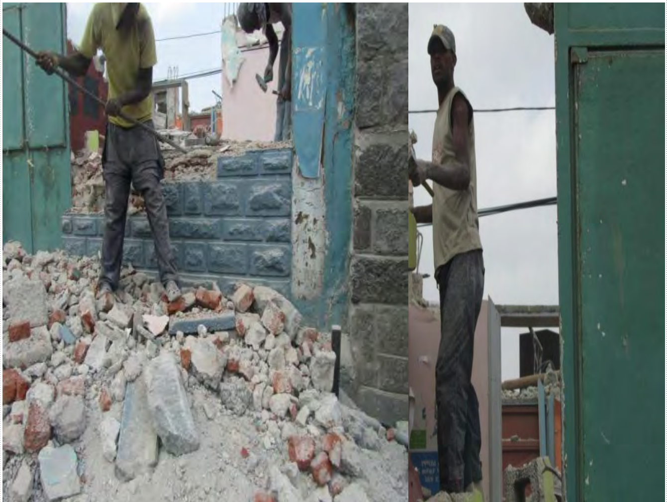
Figure 5.16: Hand demolition using hand held tools around Mexico square
