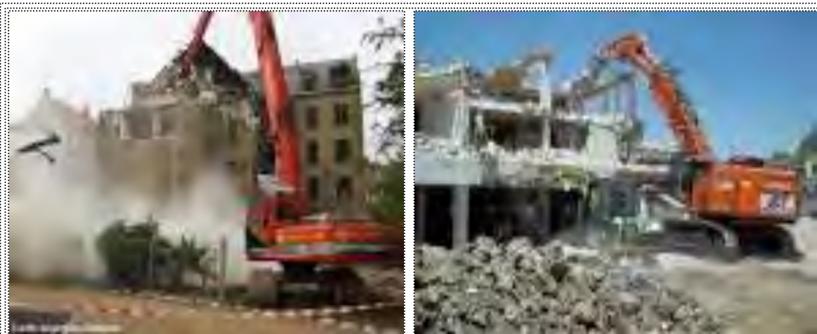
Figure 2.4: Mechanical demolitions ( jetdemolition.co.za )
