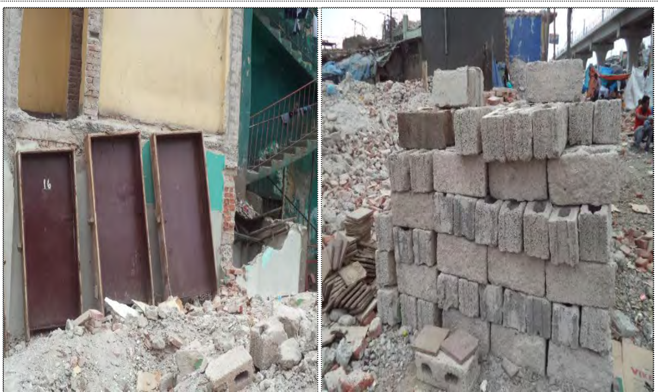
Figure 5.5: Carefully dismantled doors and hollow concrete blocks ( American Gibi )
