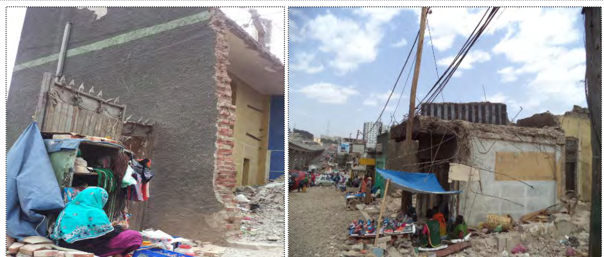
Figure 5.4: Street vendors sitting adjacent to building under demolition ( American Gibi )
