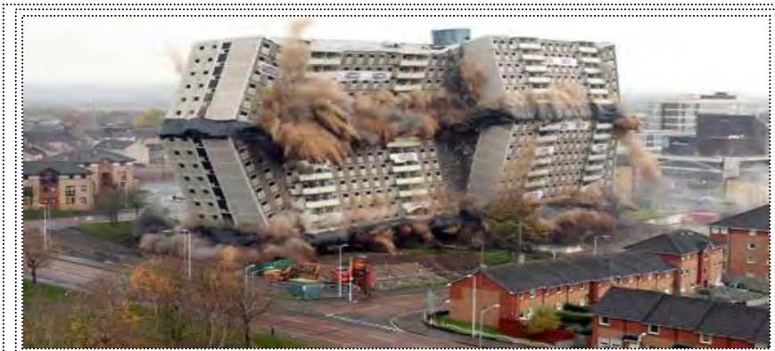
Figure 2.5: Induced collapse (Horea, 2009)
