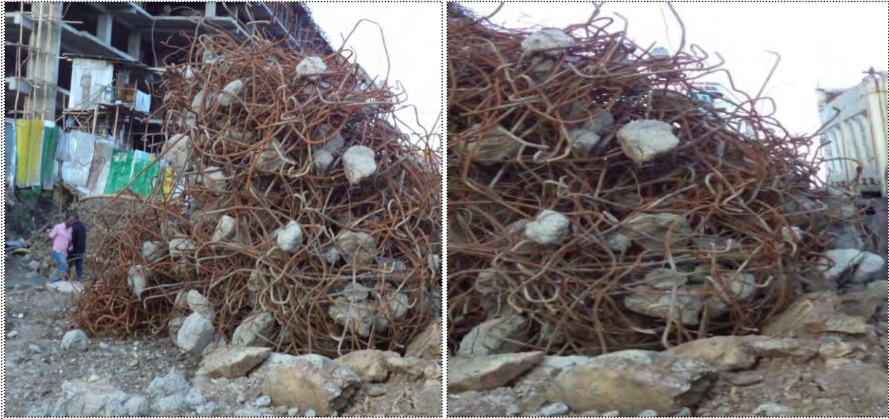
Figure 4.11: Building demolition using machine (Excavator) around 22
