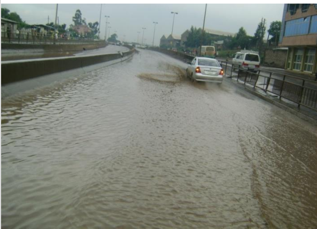
Photo 1: Storm Water pond on Ring Road (Between Kadisco-Abo roundabouts)
