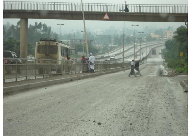
Photo 4: High speed carriageway used as bus stop (Near “Koshe” area)
