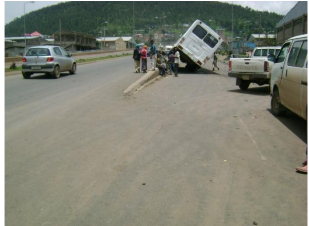
Photo 2: Accident due to invisible pavement marking (Mekanisa-Jemo road)
