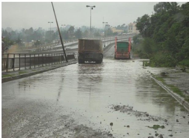
Photo 3: Outer carriageway of the Ring Road hardly functional (Near “Koshe” area)
