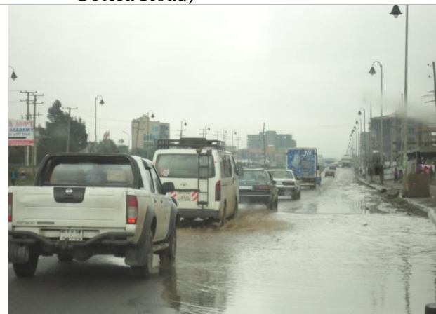
Photo 11: Two lane carriageway serving traffic as single lane (Mekanisa-Jemo road)
