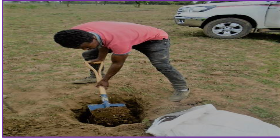
Fig 4.3 Sub grade soil sampling at station of 74+500km photo taken on May 17/2017
