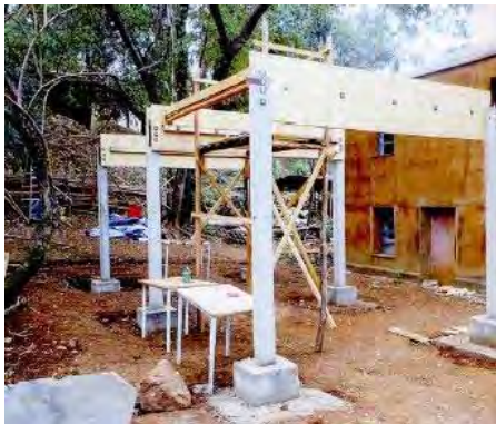
SICU prototype prefabricated concrete structure
