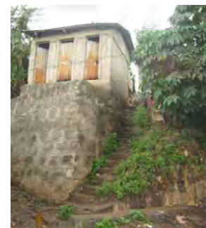
Figure 4-19: Public toilet facilities
