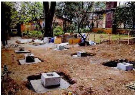
SICU prototype foundations
