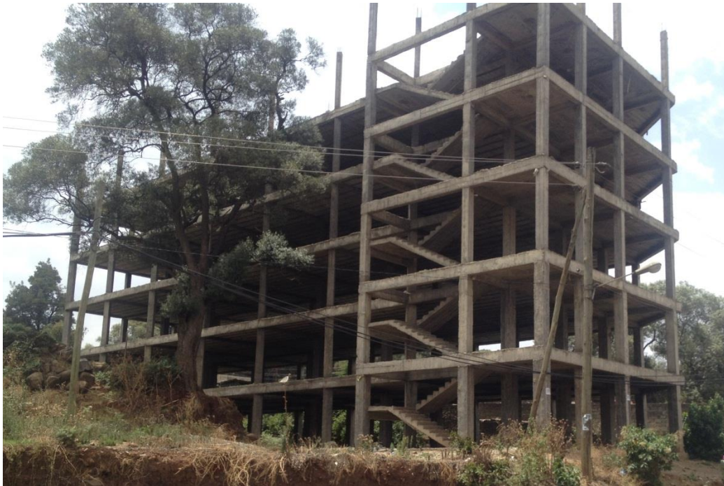
Figure 3.1 Photographic View of the building
