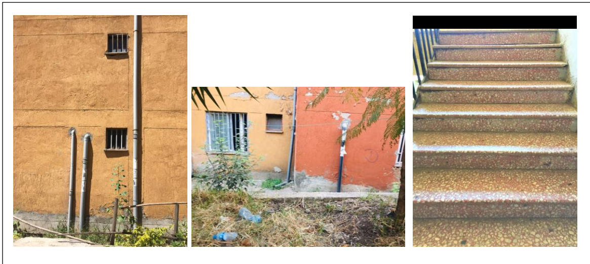
Figure 38: Individual's measure for plumbing maintenance and maintained stair case
