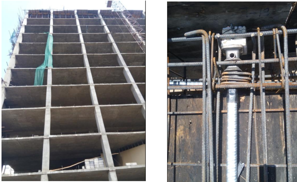
Fig. 3.2:- post-tensioned flat slab and Anchorage device at Bole around Friendship complex
