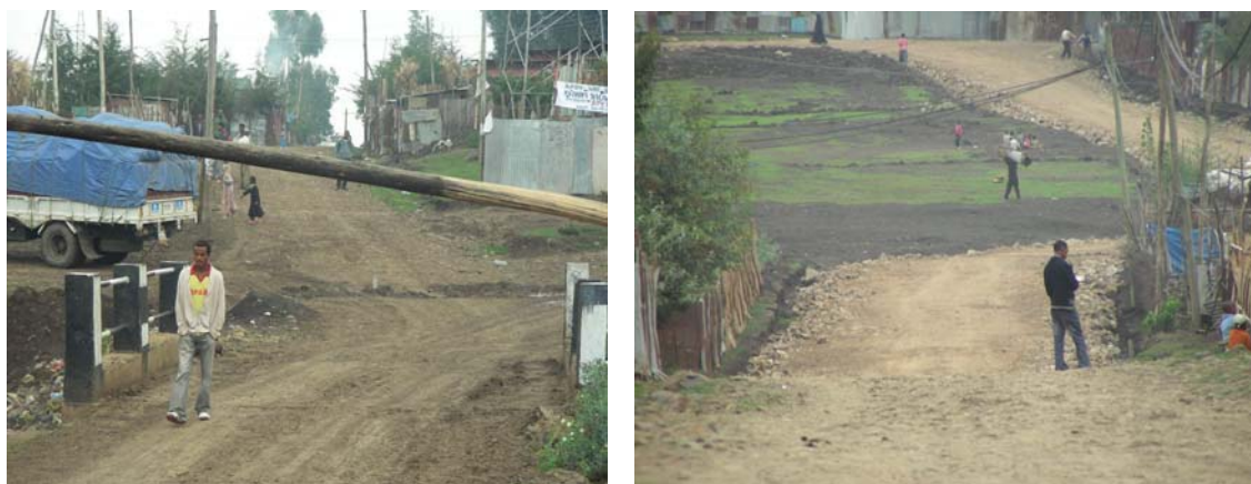
Plate 3.1 Construction of bridge and road in the study area
