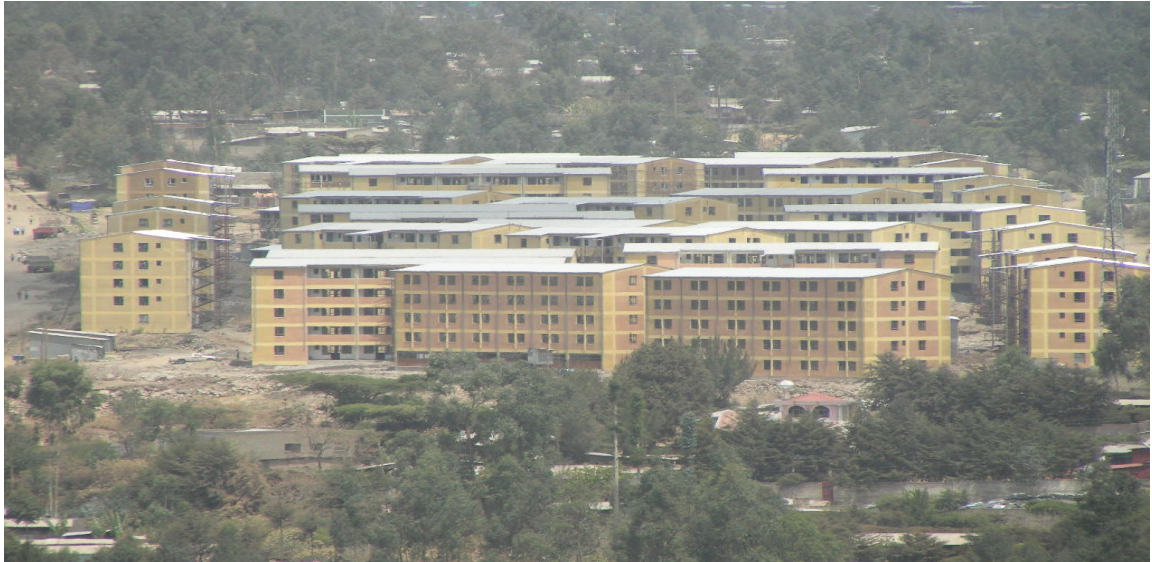
Plate 4.1 Construction of Condominium houses in the fallow land
