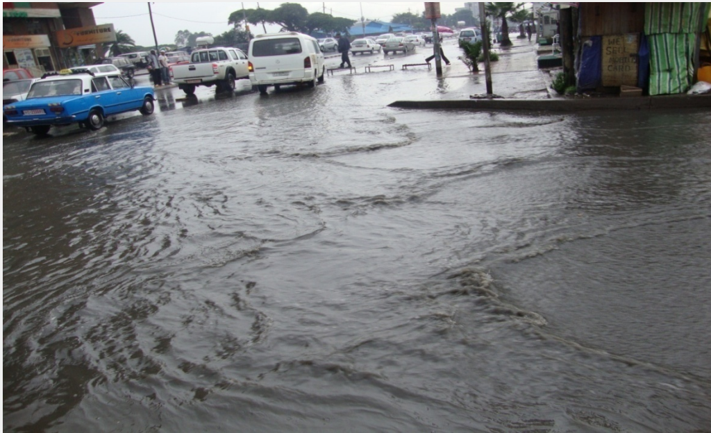
Fig1. 5 b) Congested traffic flow due to poor drainage at Gotera – Wollo sefer (August 2010)
