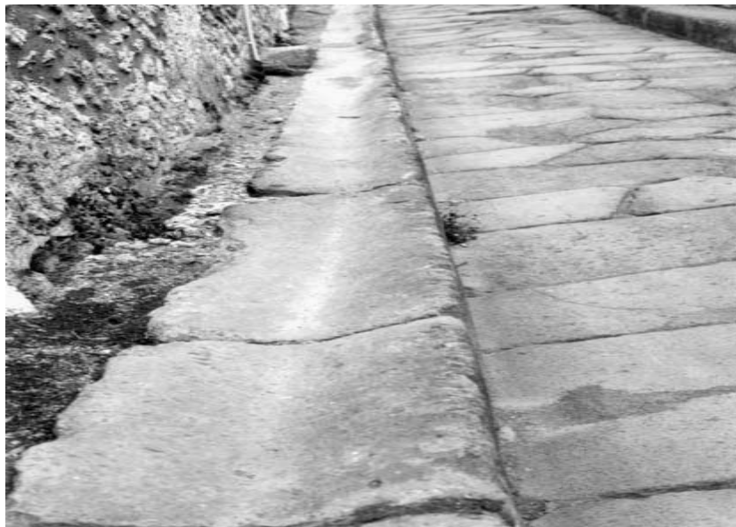
Fig 2.2 Drainage system at Pompeii (Italy) (Mays, 2004)
