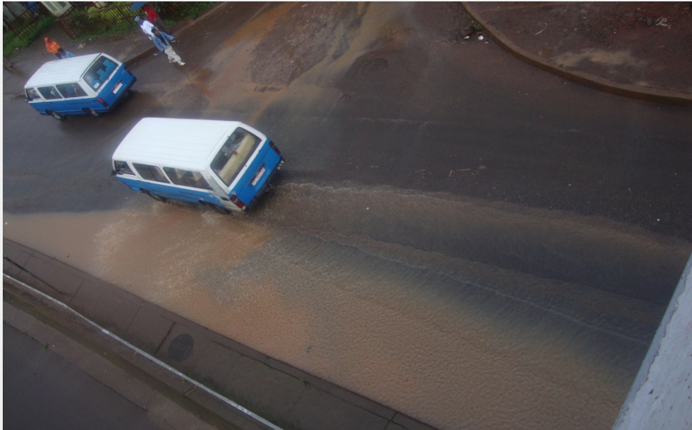
Fig1.4b) Flooding due to poor drainage problem at Zenebework (August 2010)
