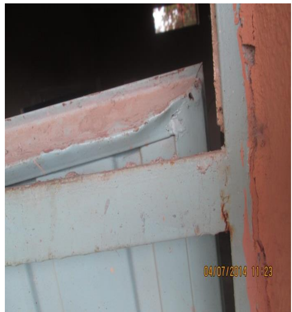
a. Doors not properly closable due to movement of wall and floor
