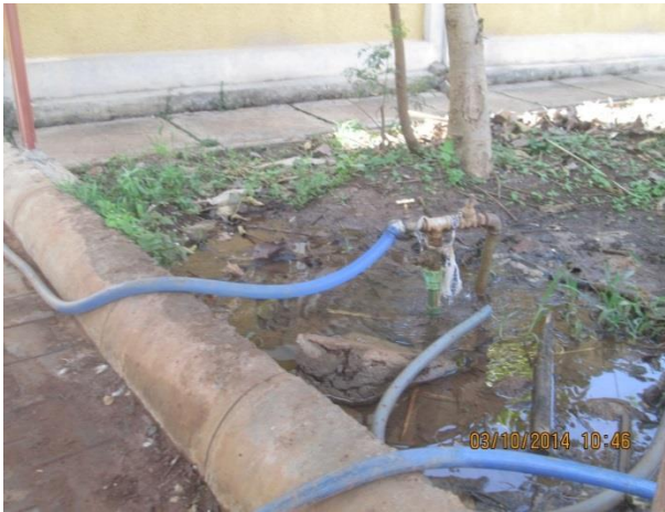
Figure 5.3 Leaking water supply pipe and damaged down pipe
