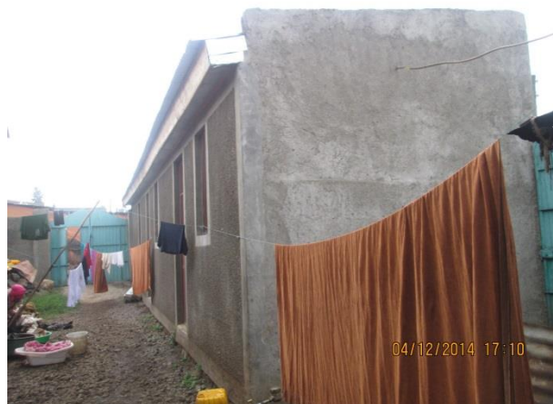
e. Masonries of most residential houses are completely covered under the soil.
