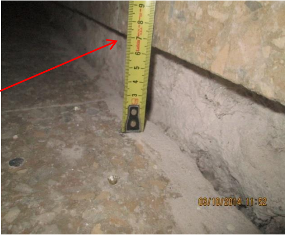
c. Floor settlement – the floor system separated from skirting by 6.5cm
