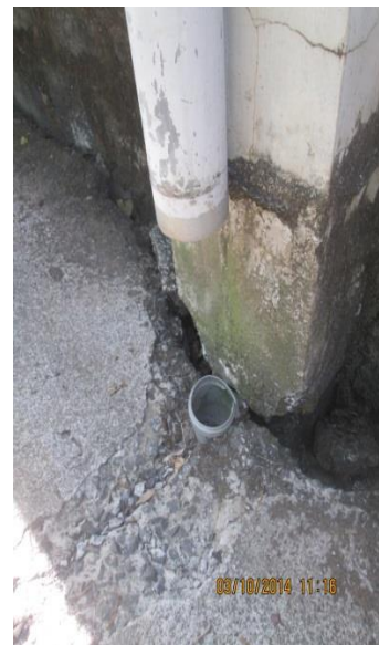
b. Walkway moved down by 47cm from its original position
