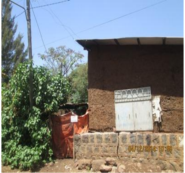
a. Masonry foundation wall partially settled around the corner due to trees/vegetation close to the building
