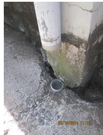
Figure 5.3 Leaking water supply pipe and damaged down pipe
