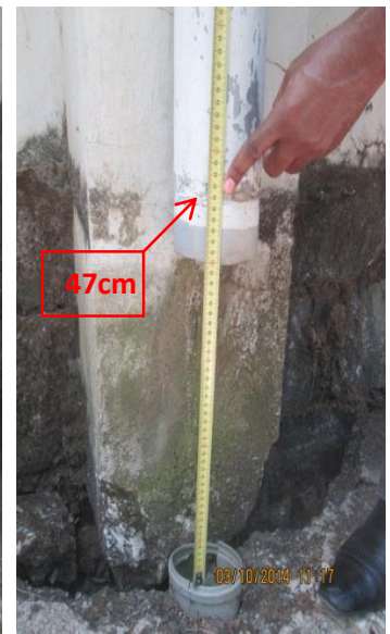
b. Walkway moved down by 47cm from its original position
