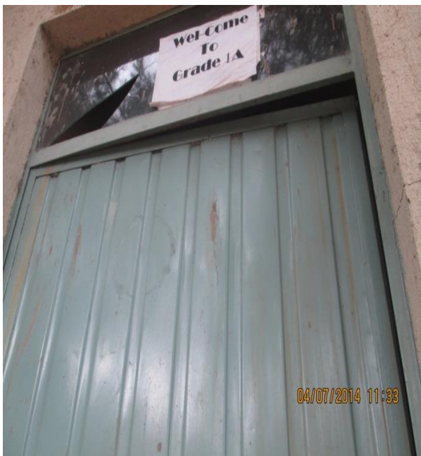
a. Doors not properly closable due to movement of wall and floor
