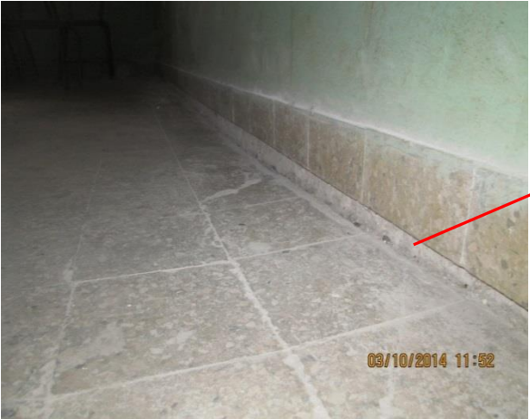
c. Floor settlement – the floor system separated from skirting by 6.5cm
