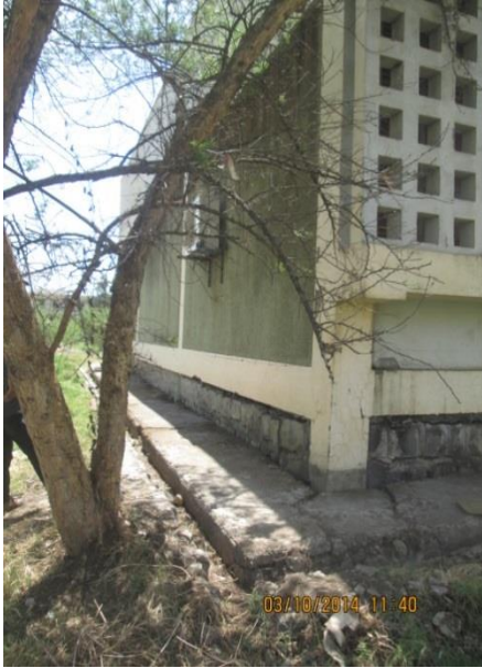
a. Masonry foundation wall partially settled around the corner due to trees/vegetation close to the building
