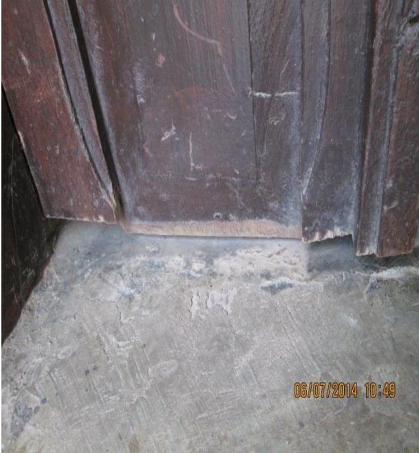
b. House owner used to cut doors at the bottom or top to adjust the stacking problem
