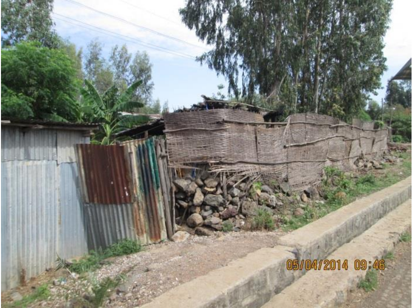
Figure 5.1 Resident areas located below road levels
