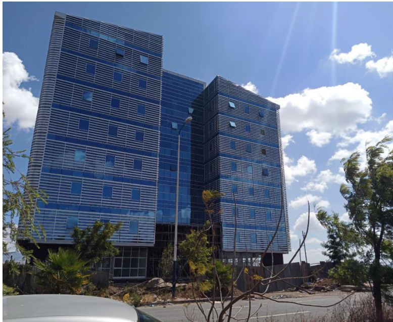
a) G+7 Prefab. Building ICT Incubation Center (2021)
