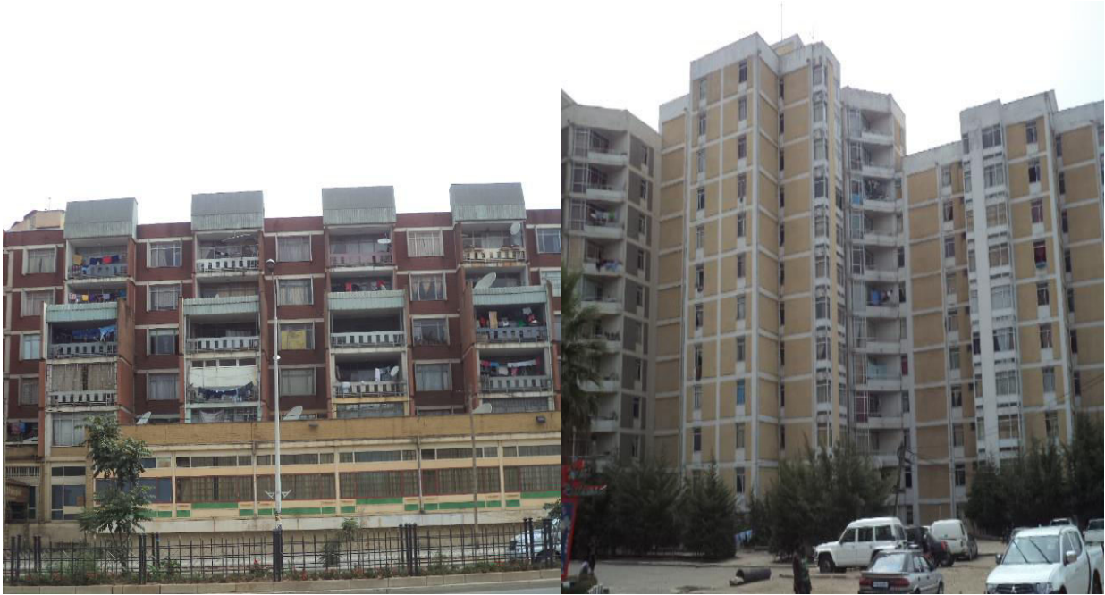
e) Bole Apartments
