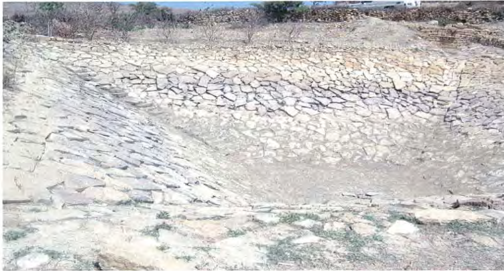
Plate 4.2: Stone covered plastic lined pond with stairs (Mai-Quiha)
