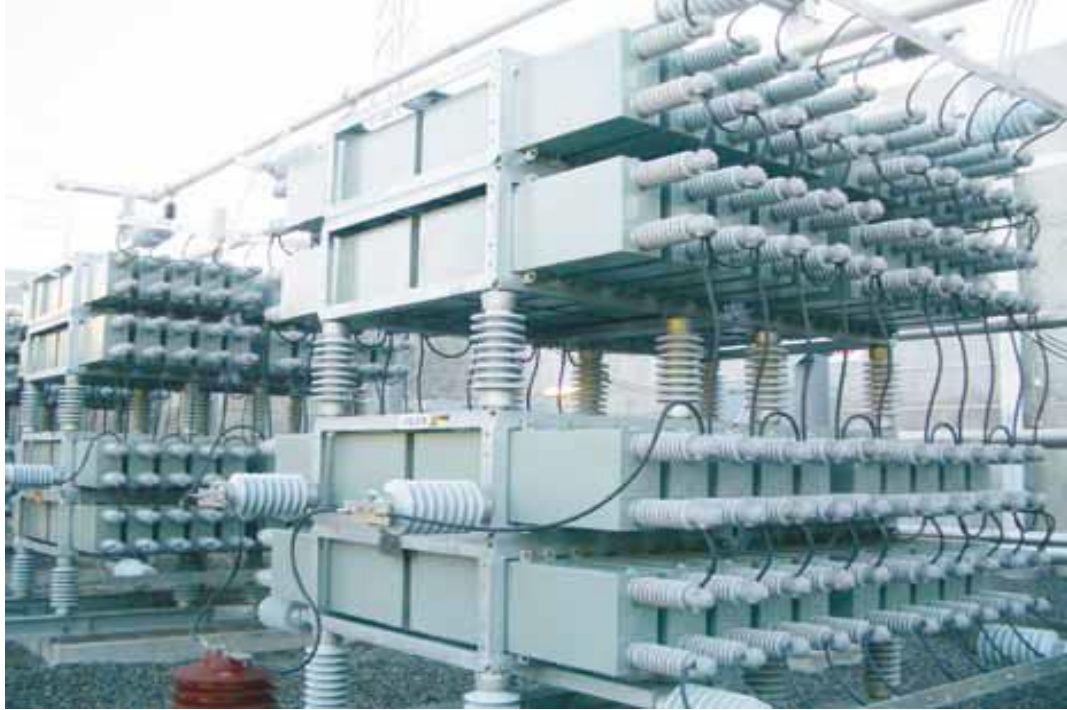
Fig2.7 Capacitor Bank in Thyristor Switched Capacitor
