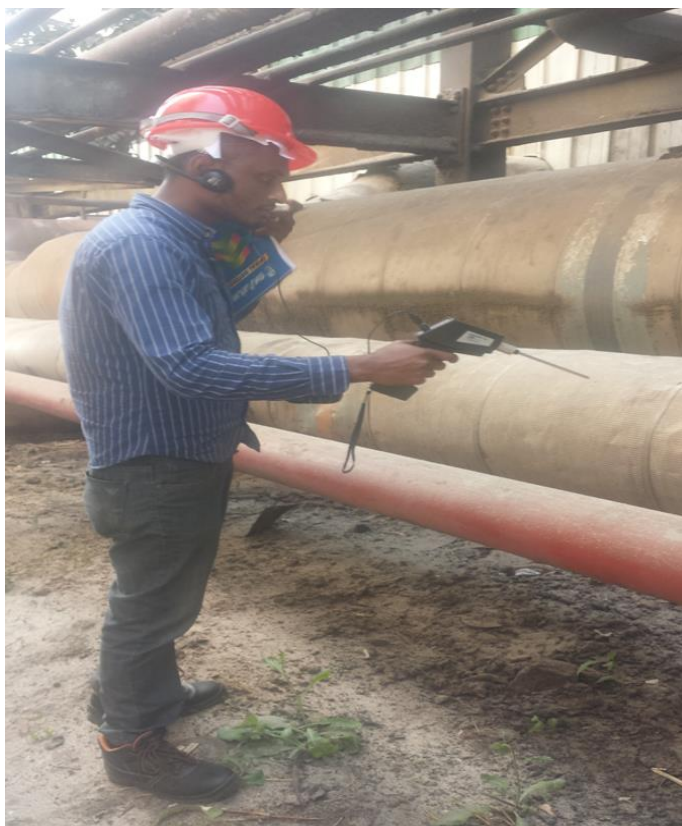
Figure 4. 10: During leak detectin using ultrasonic lead detector on steam lines
