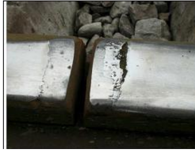
(f) Railhead spalling
