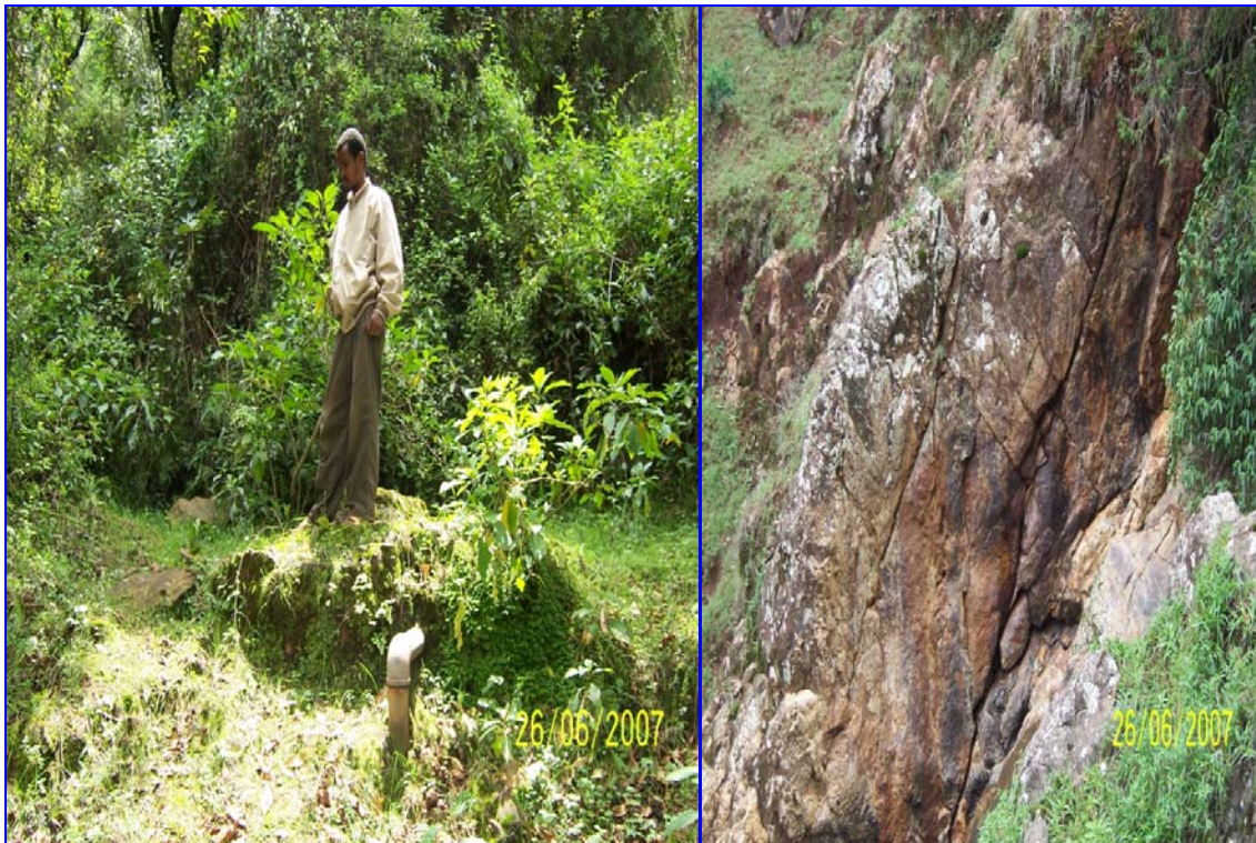
Fig 7-16: Entoto spring capping structure (left) and fractures on rhyolites around the spring (right)
