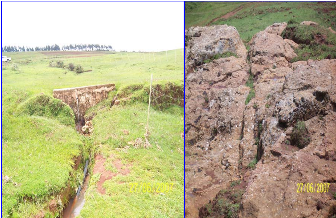
Fig. 7-10: Akako Spring capping structure (left) fractures in rhyolites around the spring.
