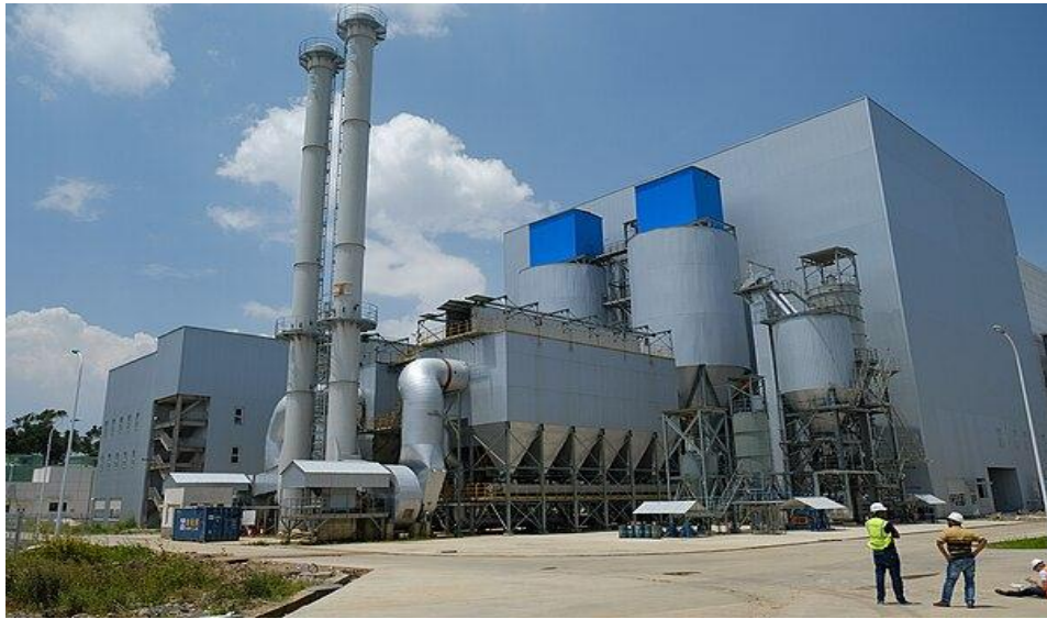
Figure 3. 3 Reppi waste-to-energy power plant
