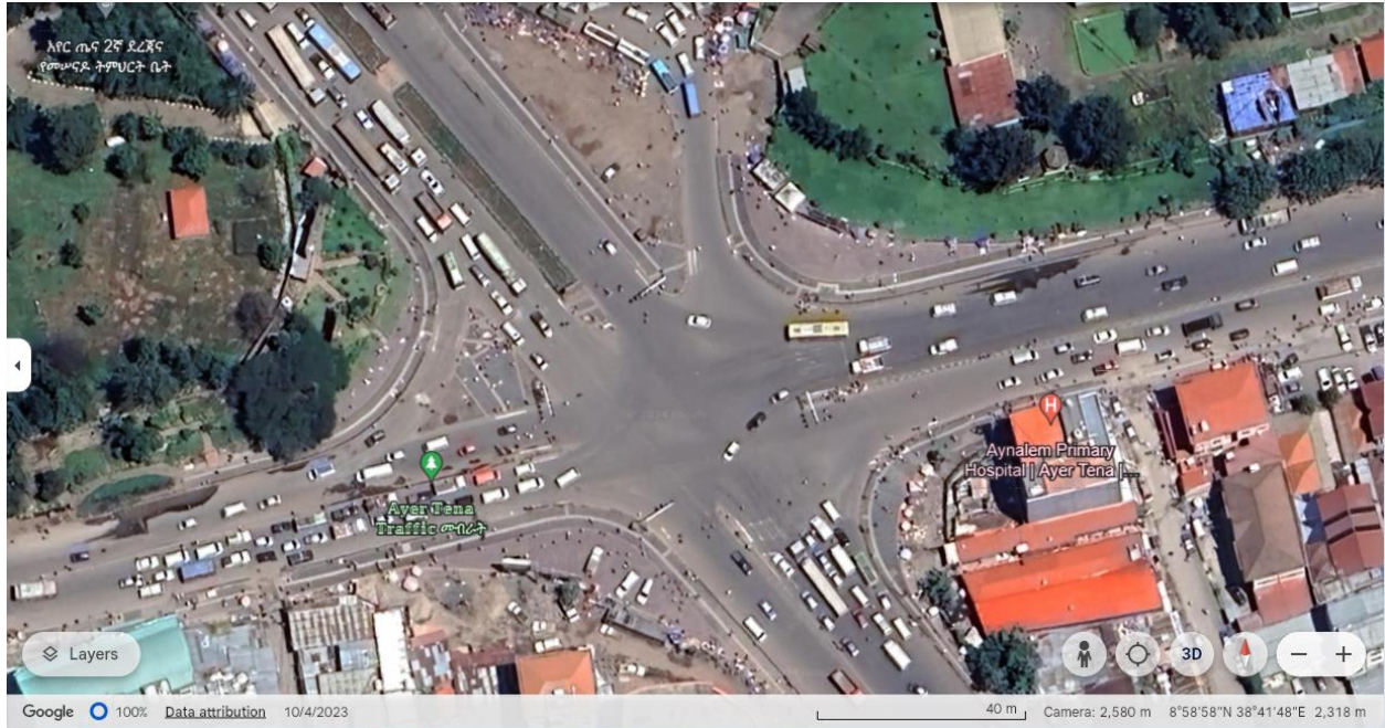
Figure 2 Ayertena Signalized Intersection
