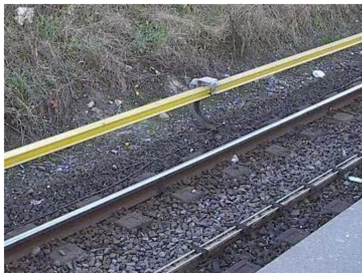
Figure 1. Third rail electrification system [1]
