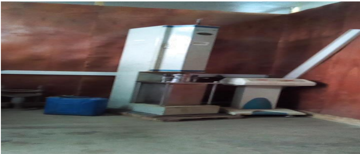
Caption 4: Compacting the mixture with Automatic Marshall Compactor
