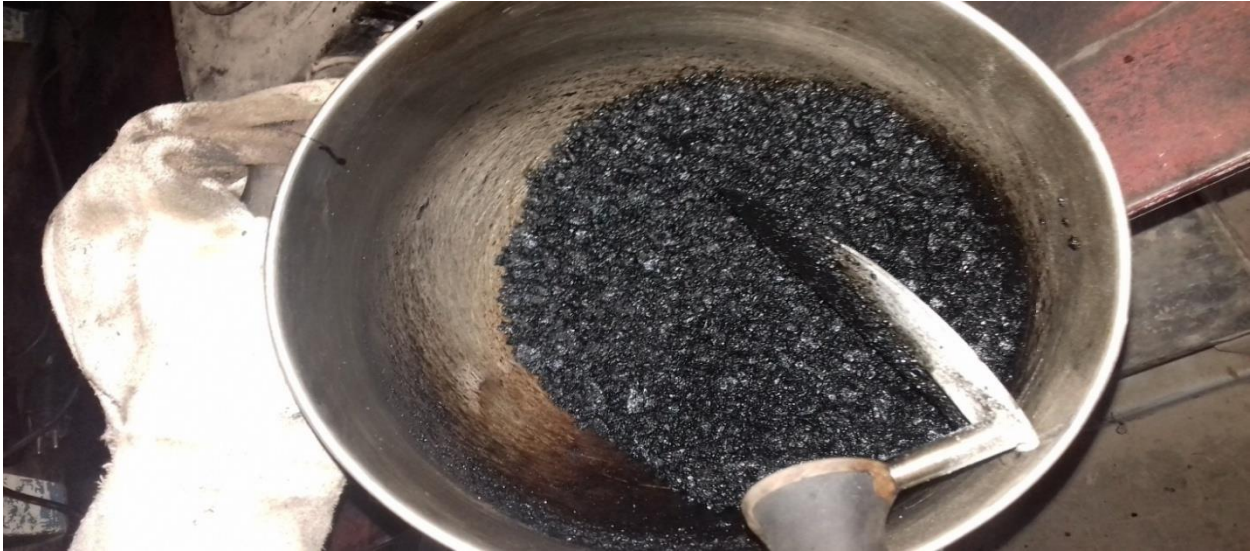
Caption 3: Mixing of aggregate and bitumen
