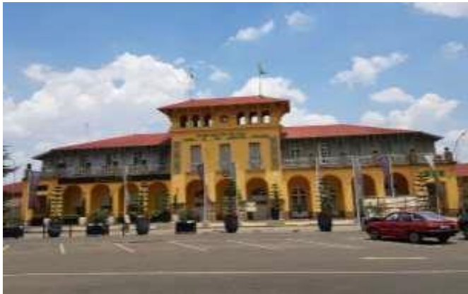
Figure 4.3. Legehar train station building from exterior
