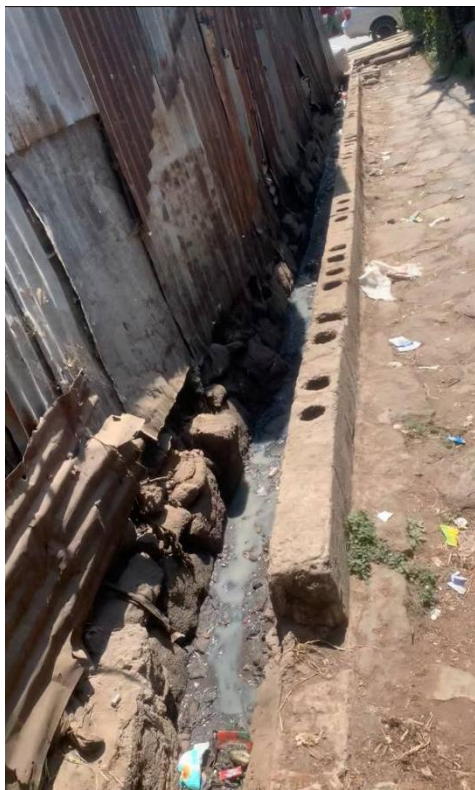
Figure 4.18. Drainage lines between houses and garbage collection
