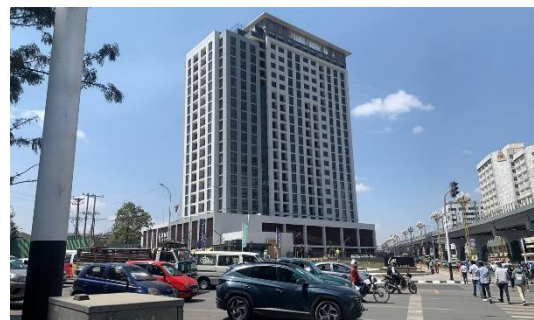
Figure 4.2. The constructed luxury apartment in the place of the shipping headquarters.
