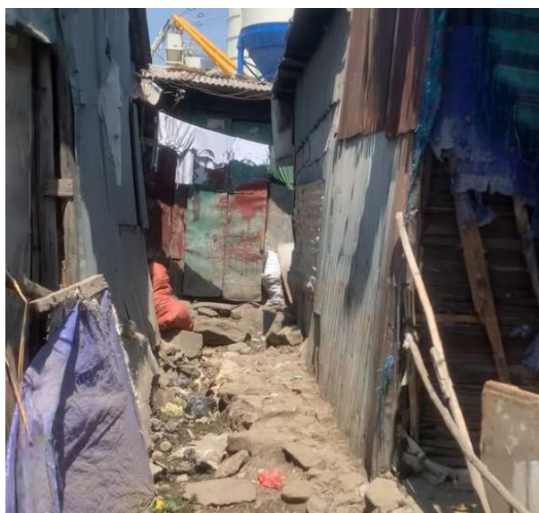
Figure 4.21. Drainage line at internal roads
