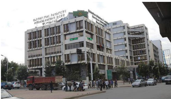
Figure 4.1. The earlier, now demolished Ethiopian shipping and logistic building
