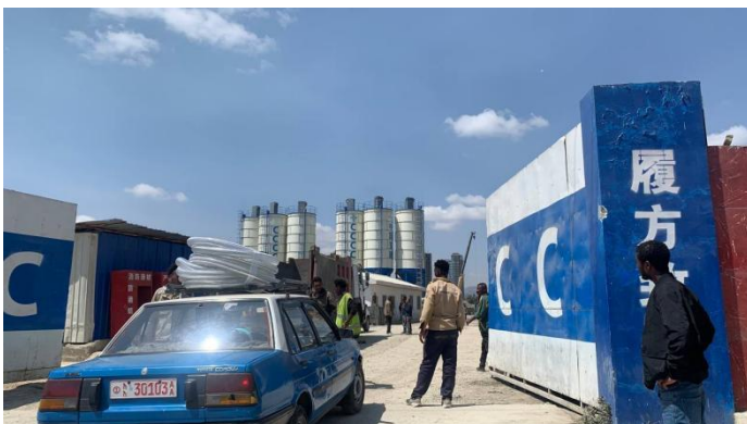
Figure 6.3. The ongoing construction site (Source: Taken by the researcher, 2025)
