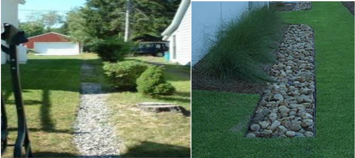
Figure 2.4: Infiltration trench (Source:Portland Water District, 2006).
