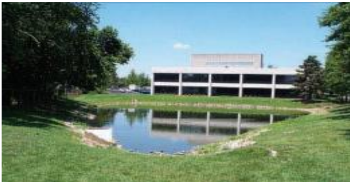
Figure 2.7: Retention pond (Source: EPA, 2009)
