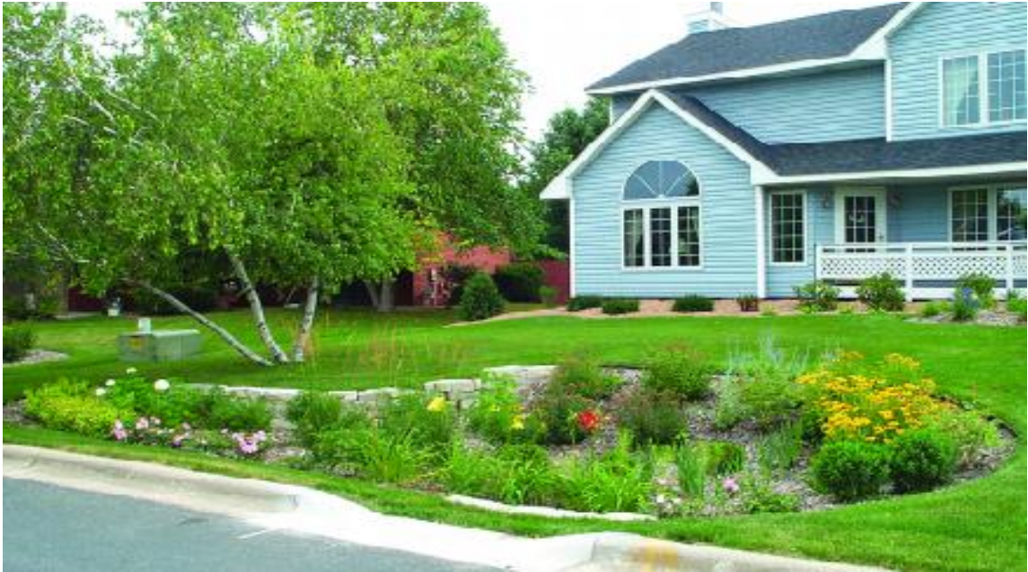
Figure 2.2: Bio-retention system (Source:NRCS, 2005)
