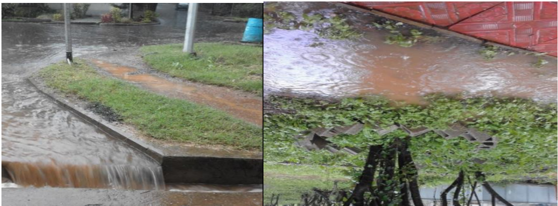
Figure 1.1: Stormwater flows from EiABC campus (Photo taken in August ,2017).
