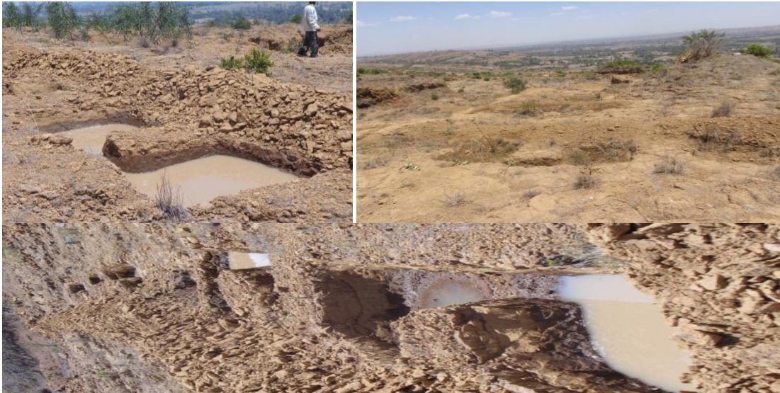
Figure 8 Stone bunds embankments and Cutoff drains
