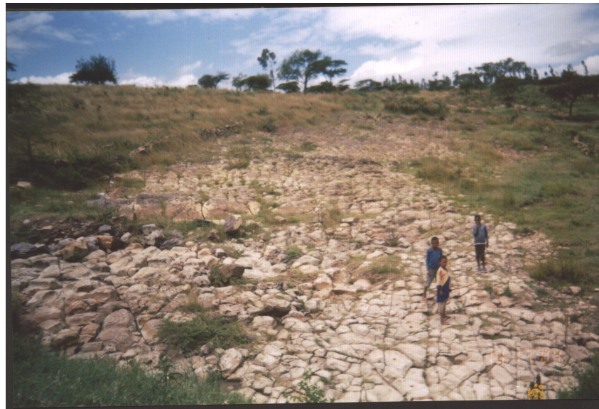
Figure 5.1 Bed rock exposed due to sheet erosion
