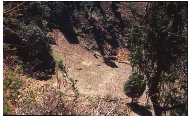
Figure 7.2 Landslide scar that damage property
