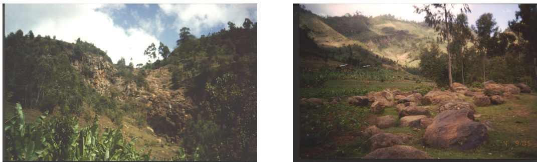
Figure 7.7 Rock fall on Damot Mountain
