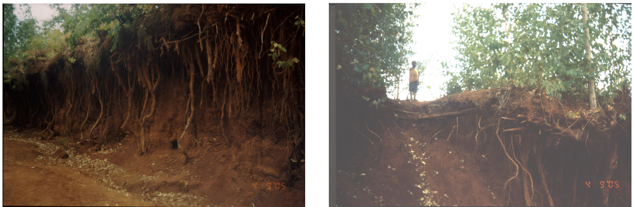
Figure 6.9 Land degradation aggravated by road cut
