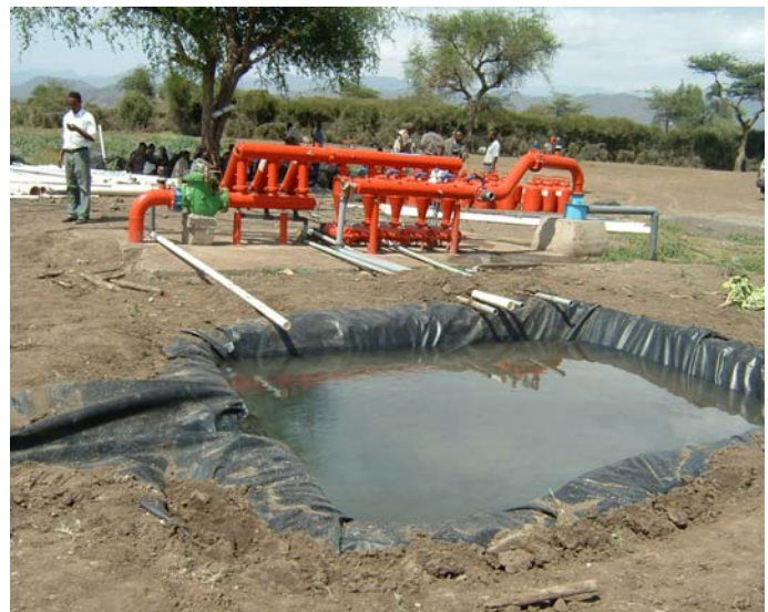
Figure 26 Well development at the valley
