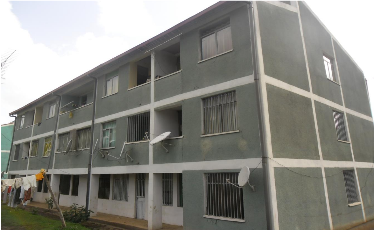
Figure 6: One of condominium building in hosanna town
