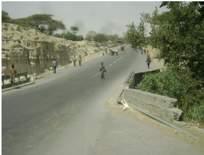
Figure 12. Photo showing Bulbula River Bridge, Modjo side approach
