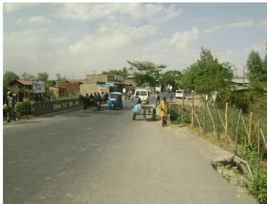
Figure 1: Meki Bridge accommodating motorized as well as non-motorized users .
