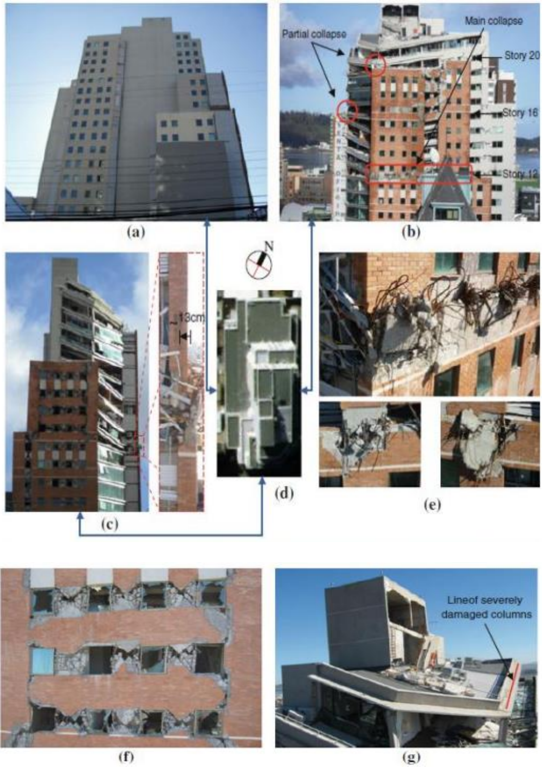
Figure 2.1 Overview of building TO-9:
