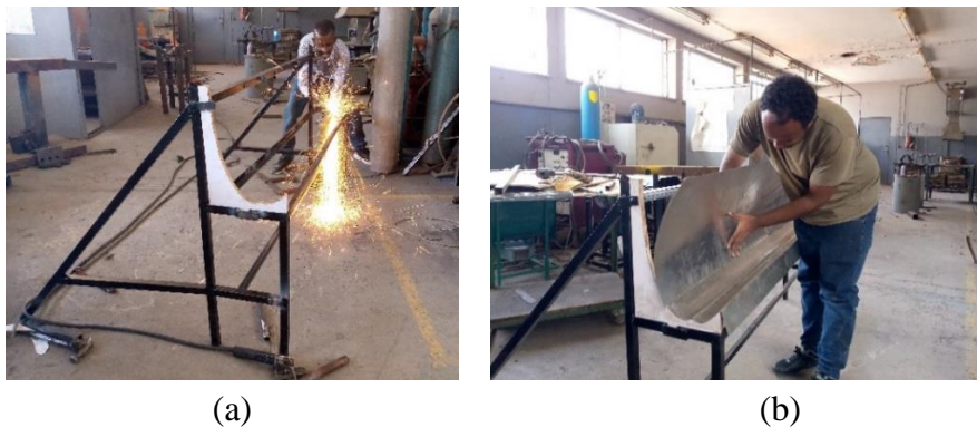
Figure 5-2: Photographs of fabrication stages of the supporting structure
