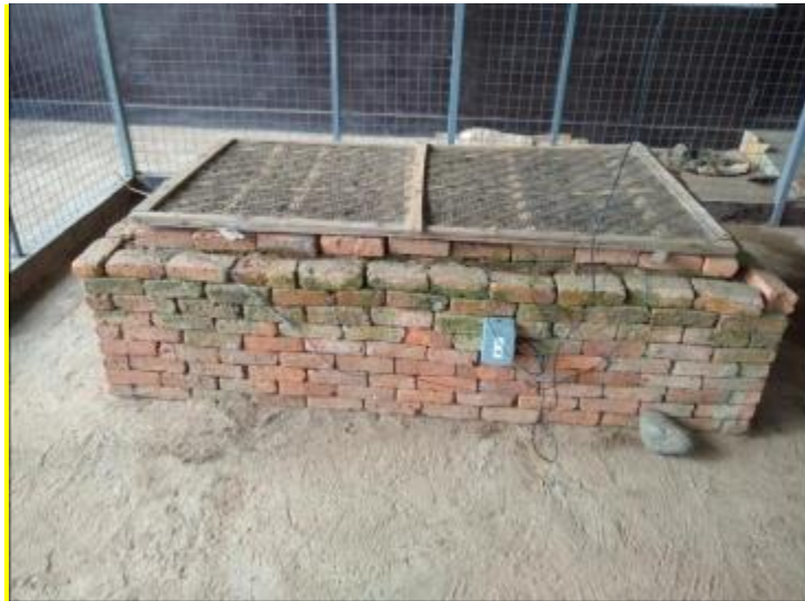
Figure 2. 2: A brick zero energy cooling chamber (ZECC) (Ambuko & Wanjiru, 2017).
