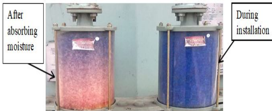
Figure 2.5: Color of silica jelly before and after absorbing excessive moisture
