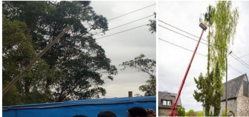
Figure 2.1: Tilted pole (left side) and a tree risk for distribution system (right) (Source: photo from the study area (left side) and website (right))
