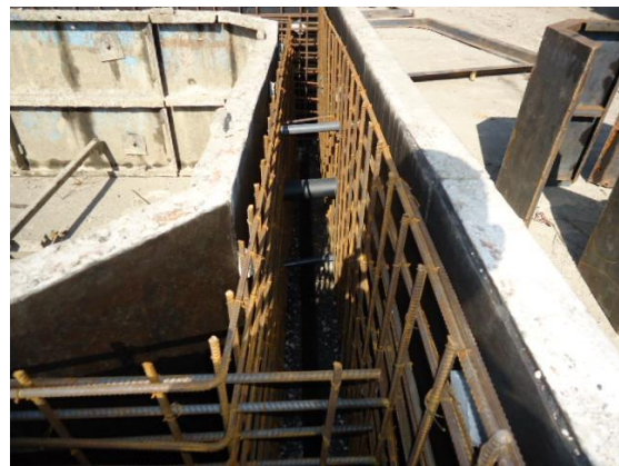
Figure 4-2: Reinforcement bar within assembled Mould
