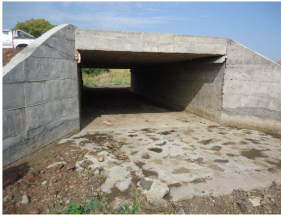
Figure 2-4: RC Box Culvert;
