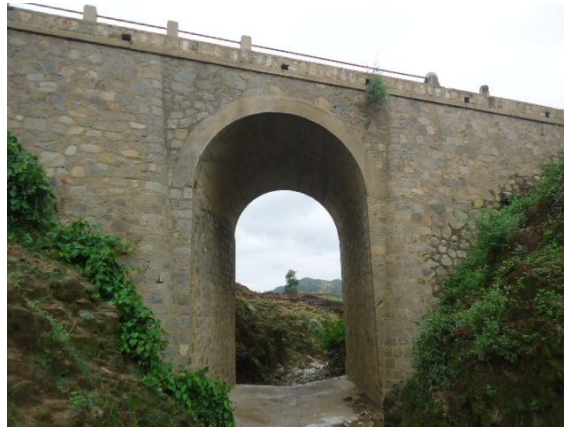
Figure 2-1: Masonry Arch Culvert
