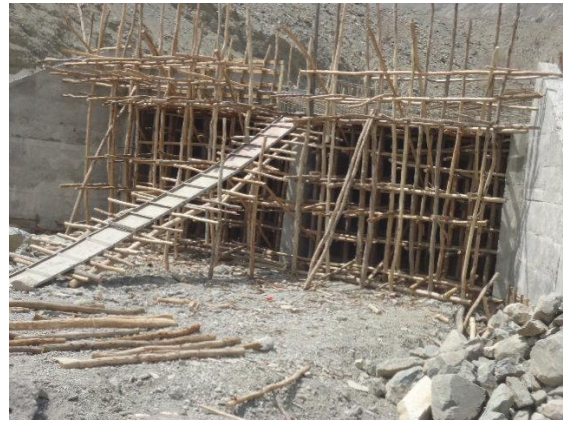
Figure 4-4: Falsework, formwork and reinforcement work completed and ready for concrete casting
