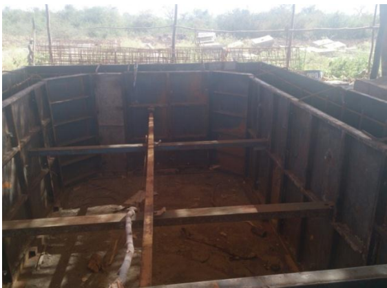
Figure 4-1: Steel Formwork Prepared before Concrete Casting
