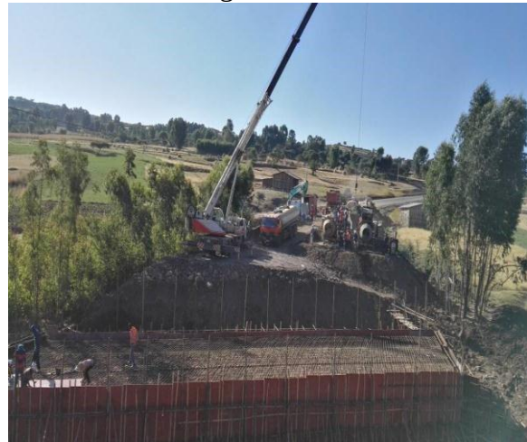
Figure 4-6: Machineries and materials prepared for top slab concrete casting
