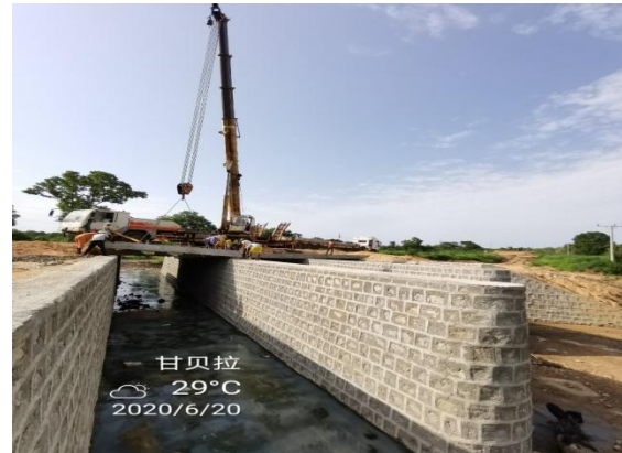
Figure 4-2: Installation process of precast slab
