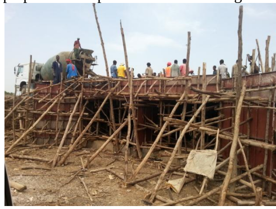
Figure 4-8: Concrete casting process for top slab of box
