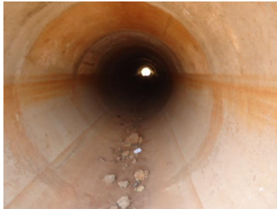
Figure 2-2: RC Pipe Culvert
