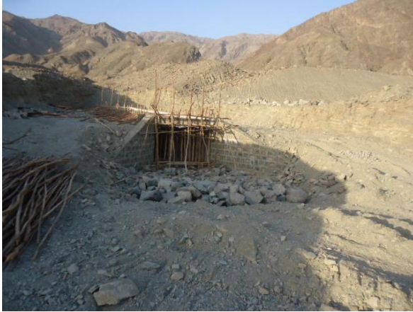
Figure 4-1: Falsework and Form Work Arrangement
