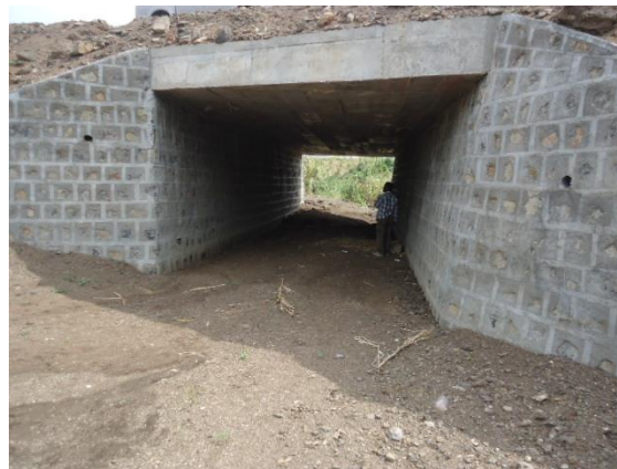
Figure 2-3: Slab Culvert
