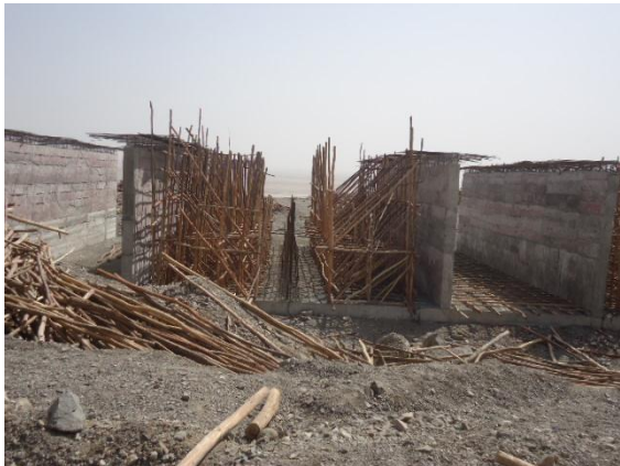
Figure 4-3: Falsework preparation activity for top slab of box culvert
