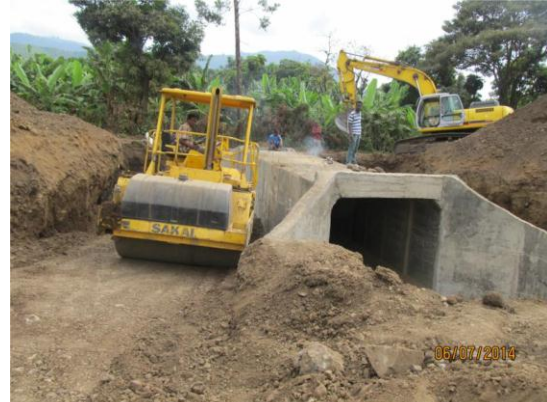
Figure 4-6: Backfilling activity which begin immediately after installation
