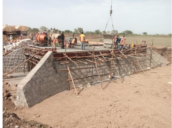
Figure 4-2: Concrete Casting Process
