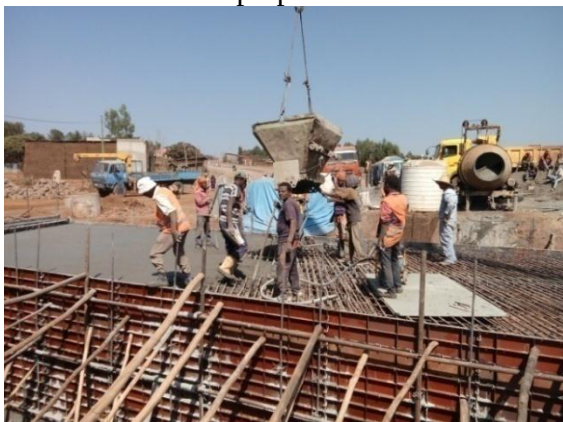
Figure 4-7: Concrete casting process for top slab of box
