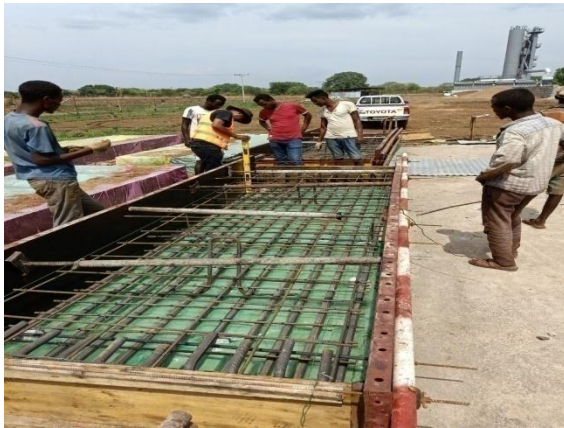
Figure 4-1: Steel Form Work and Reinforcement bar arrangement
