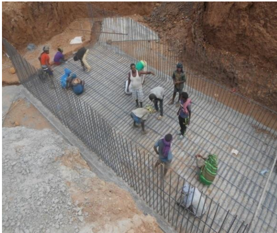
Figure 4-5: Bottom slab and wall reinforcement bar preparation work
