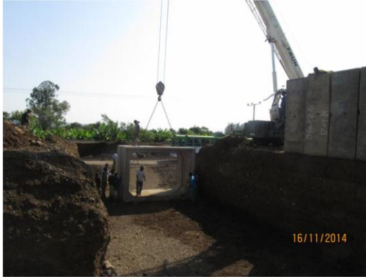
Figure 4-5: Installation process of precast Box
